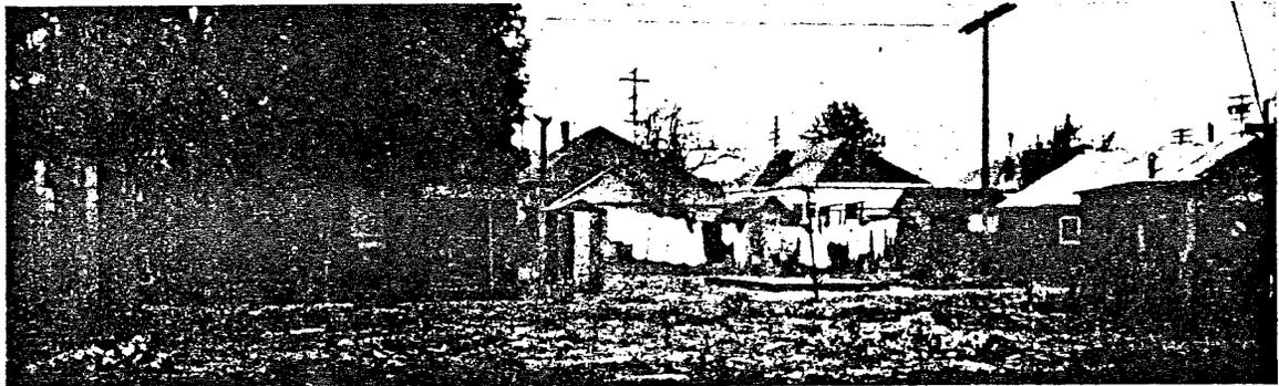
PHOTO 29 - Same location as Photo 28, showing three outdoor privies which serve whole Housing Unit. These are not fly-proof and are swarming with flies.
