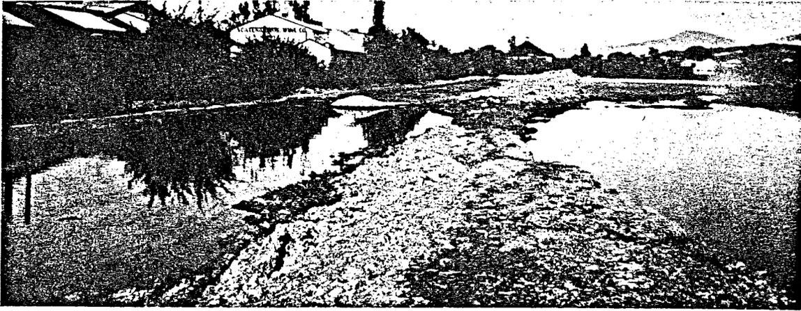
PHOTO 14 - Effluent pond Healdsburg Dehydrating Plant, processing potatoes and carrots. High organic content and very odoriferous. Pond on left has overflowed onto field at right.
