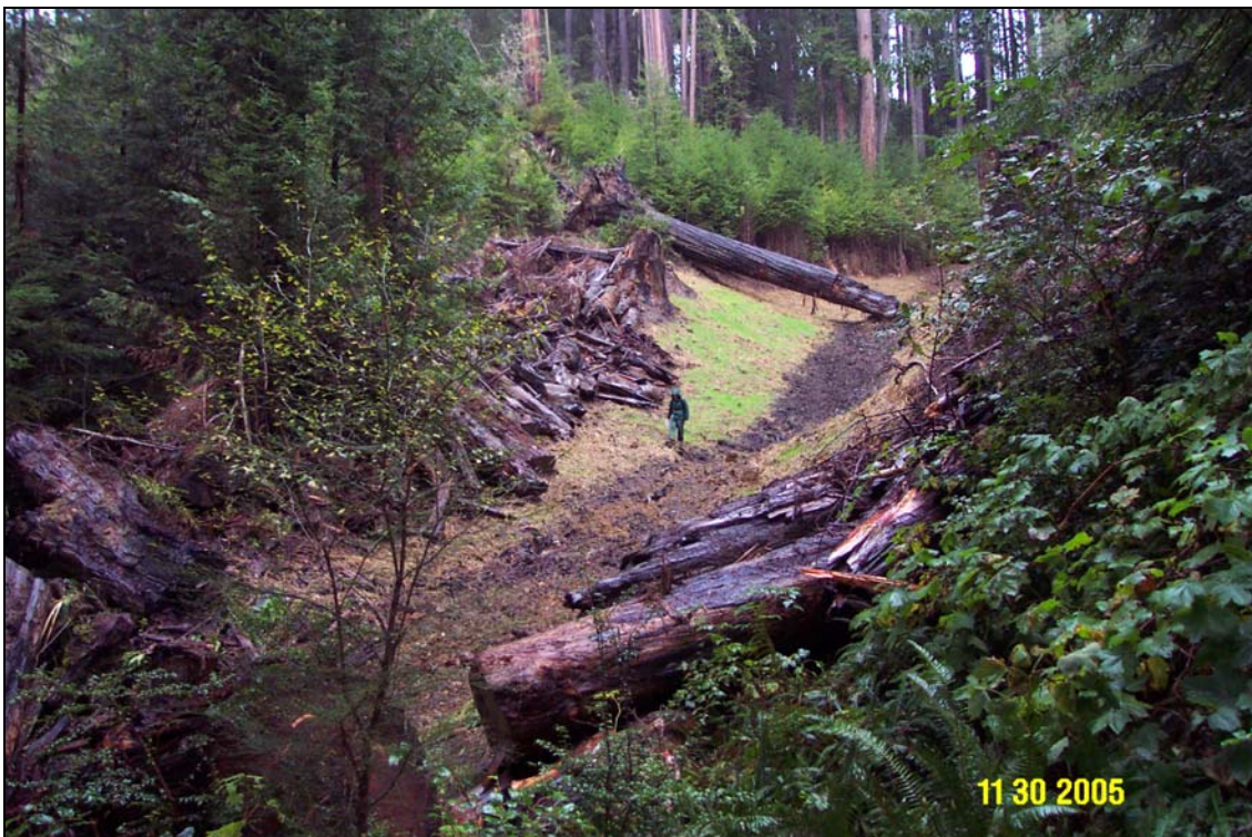
Photos 9A and 9B. R14 Road, site #145, pre and post treatment. View is approximately from the bottom of the excavation. Note the large old growth tree that is resting in the upper portion of the site. The tree had fallen prior to decommissioning activities due to a cutbank slide on the side of the crossing. Note the person, located in the center of the bottom photo, for scale.
