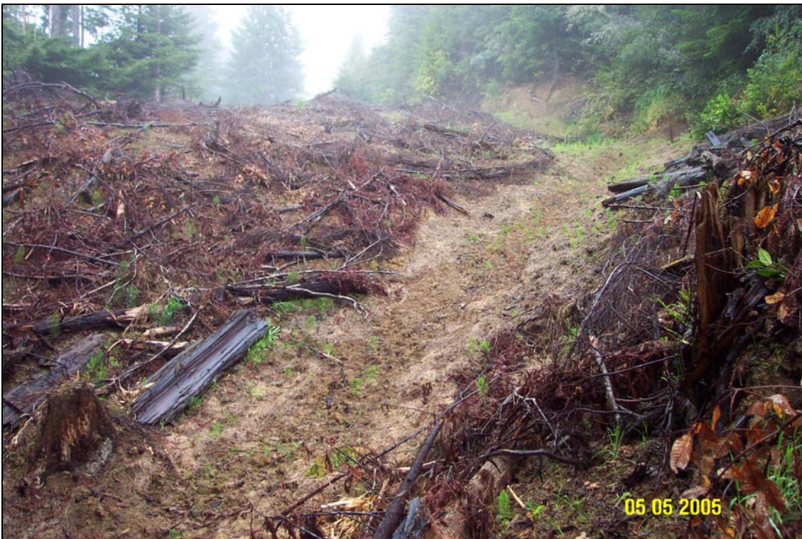
Photo #4. The same stream crossing as it looked after going through one winter. The view is from the lower end of the excavation looking upstream to the top.
