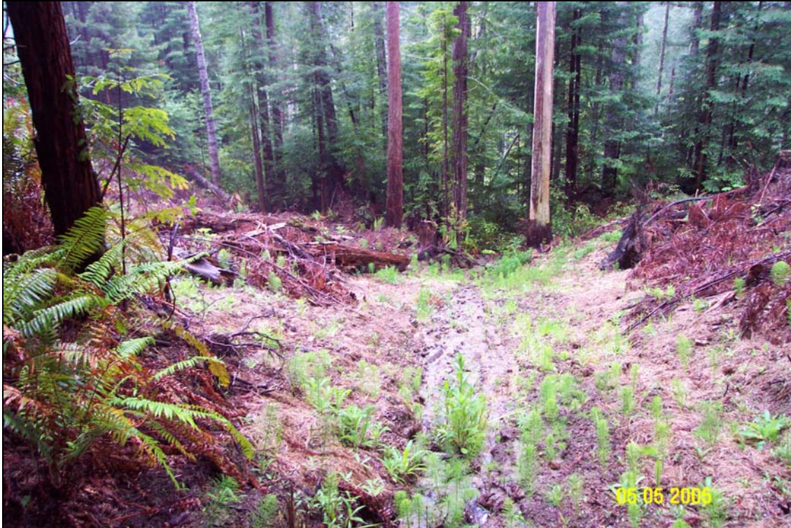
Photo #6. Site #3, U06.6966 Road, post-treatment. View is from the top of the excavation looking down to the bot. This picture was taken in May, 2005 after the site had gone through it's first winter, post treatment. The channel is showing almost no signs of adjustments.
