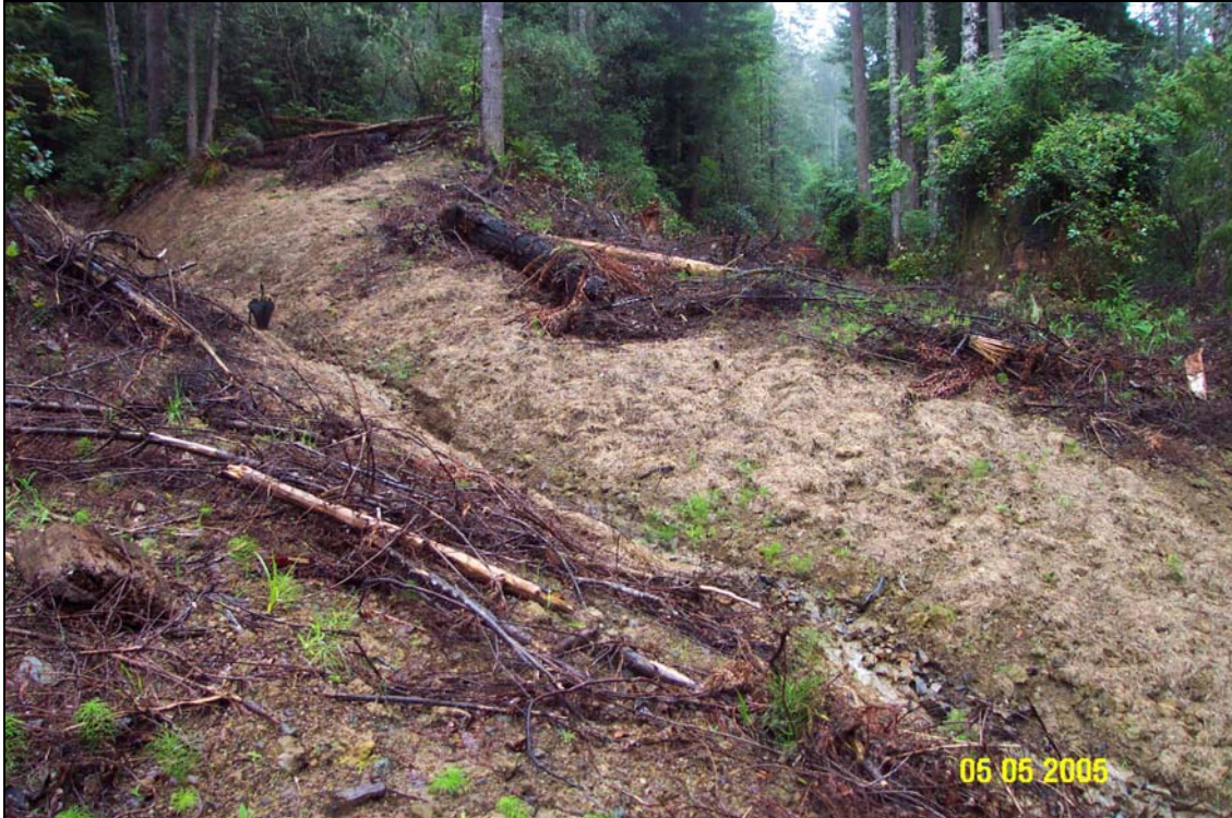
Photo 6. Stream crossing Site #17 approximately one year after decommissioning. View is similar to the photo above and was taken from above the right side slope near the middle of the excavation looking toward the slash covered left road approach. The upstream end of the excavation is in the upper left corner of the photo.
