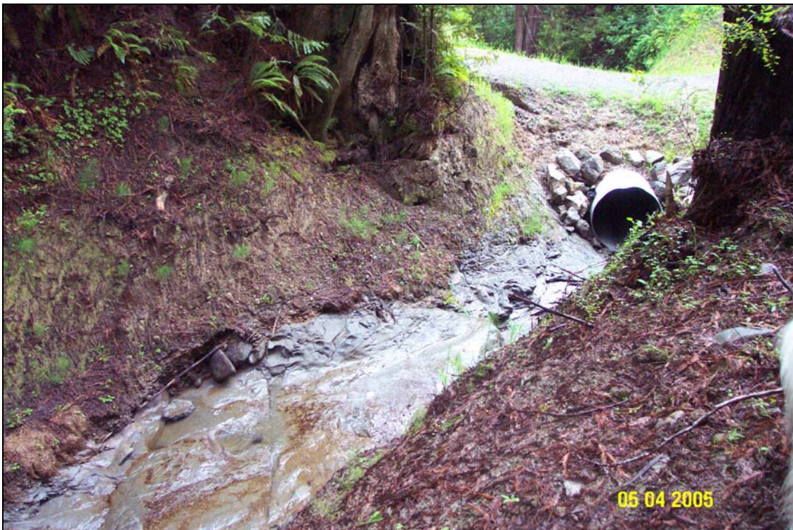
Photos 8 and 9. U06 Road, site #1129, post-treatment. Top photo show picture of the upstream extent of the channel excavation upstream from the crossing. The bottom photo shows part of the excavated channel as well as the new culvert inlet in the upper right of the photo. Both photos show the gray, slick surface of the Wildcat siltstone bedrock which controlled the depth of the channel excavation.
