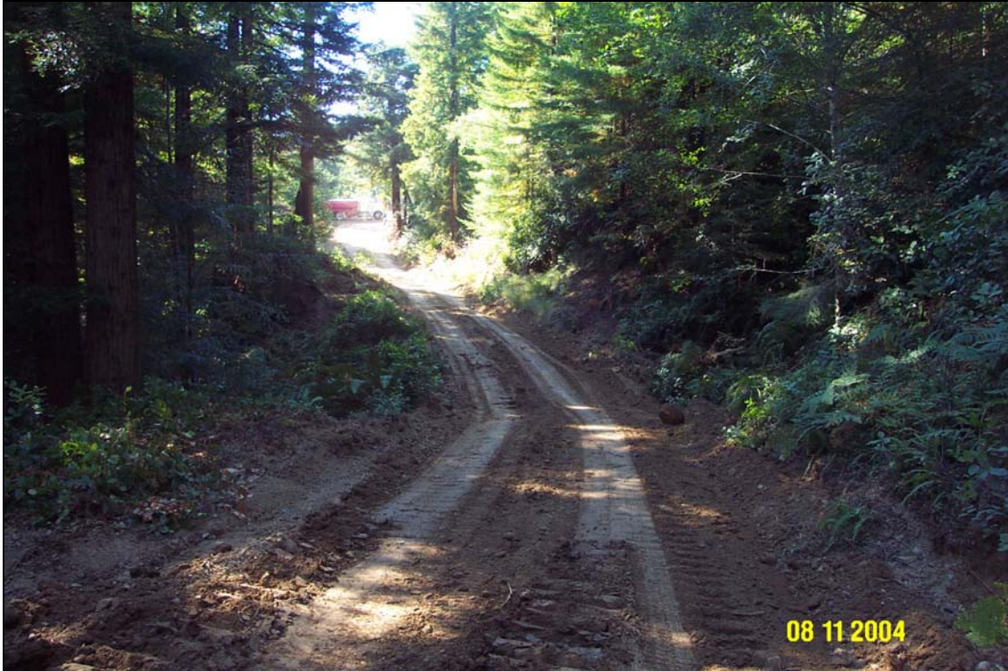
Photo #19. Site #8, stream crossing on the U06.6966 Road, pre-treatment.
