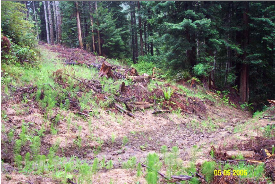
Photo #16. Another shot of Site #6, U06.6966 Road, post-treatment after one winter. View is from the right side slope near the top, looking downstream toward the bot.
