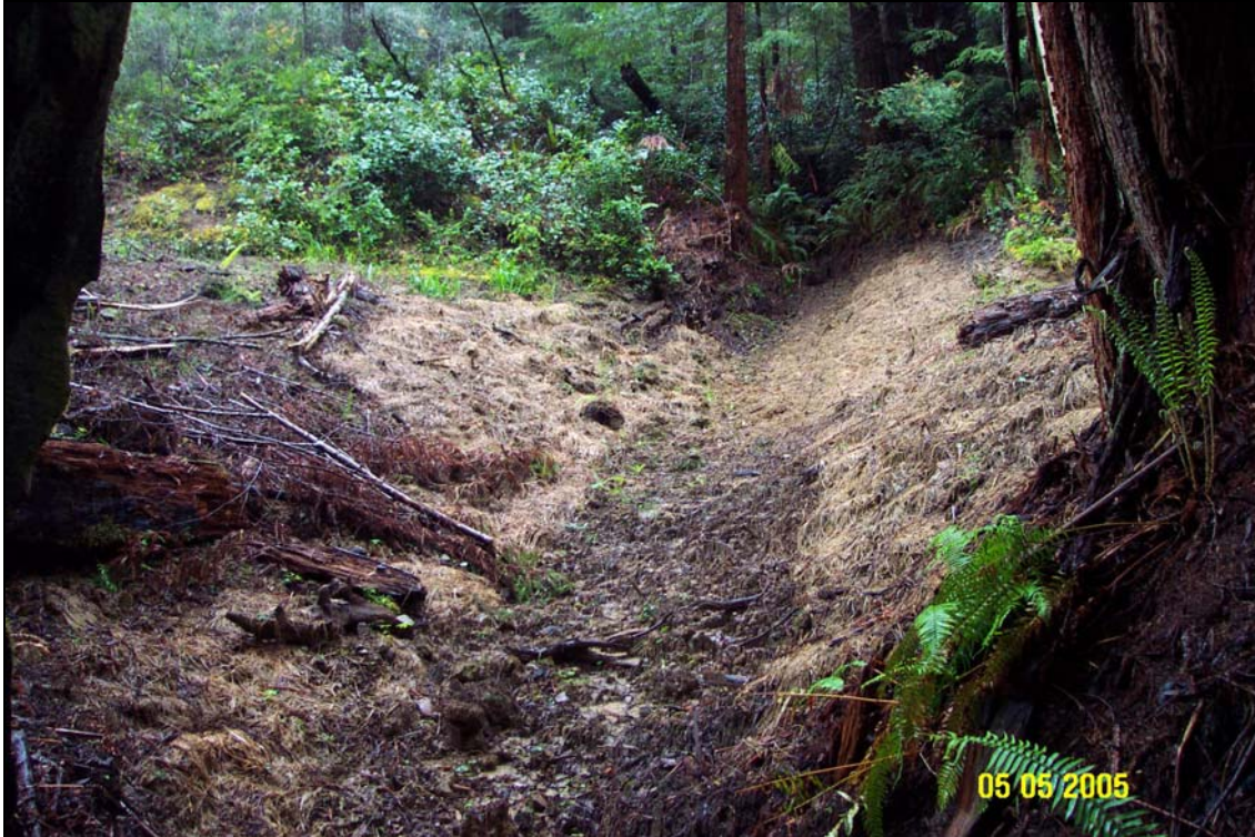
Photo #21. Site #8, stream crossing on the U06.6966 Road, almost one year after treatment. Picture taken from near the bot looking upstream. The new stream channel shows very little signs of adjustments.
