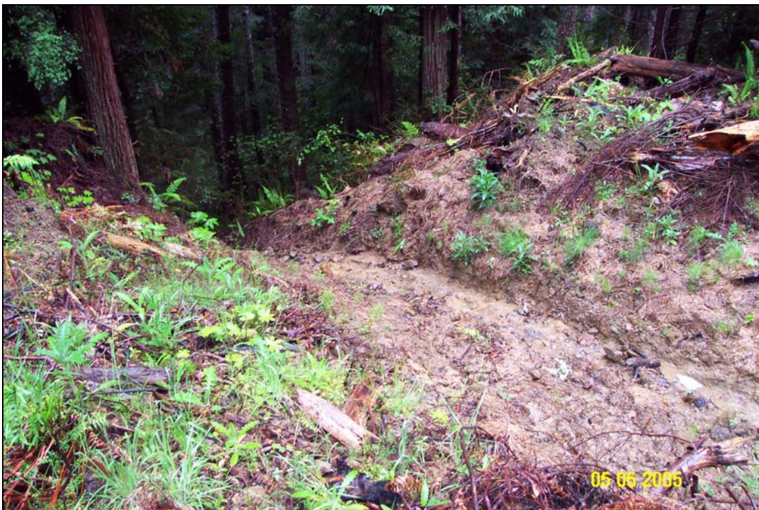
Photo #17. Site #6, post-treatment after one winter. View is from the left side slope near the lower end of the excavation, looking downstream toward the bot. Note the convex upward shape of the channel bottom as it approaches the bot, generally not the shape that is desired. A straight line or concave upward profiled is preferred, removing all fill. In this case, the excavator hit bedrock which controlled the resultant profile and should likely result in minimal channel adjustments.
