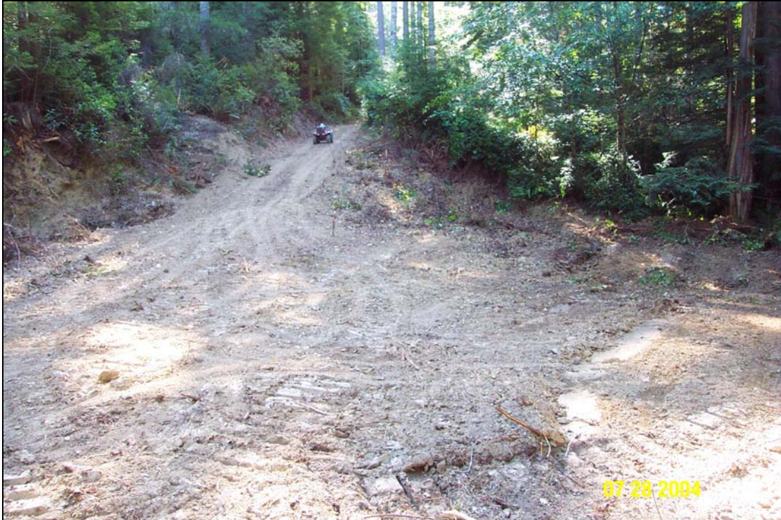
Photo 5. U06.6966 Spur 1 Road, Site #17, stream crossing, pre-treatment. The picture was taken from the right side of the terminal landing on this road that buried the original stream valley. The downstream end of the crossing is on the right side of the photo. Note the quad in the top center-left of the photo on the left road approach.
