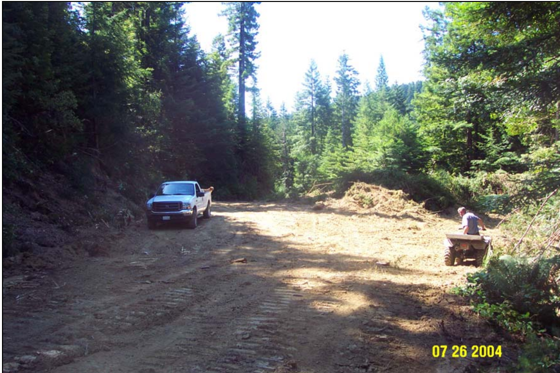
Photo #1. Site #1, U06.6966 Road, pre-treatment. Landing buried stream valley which had actively enlarging sinkholes. Site #2, another stream crossing, is located on the far side of the landing near the center of the photo.
