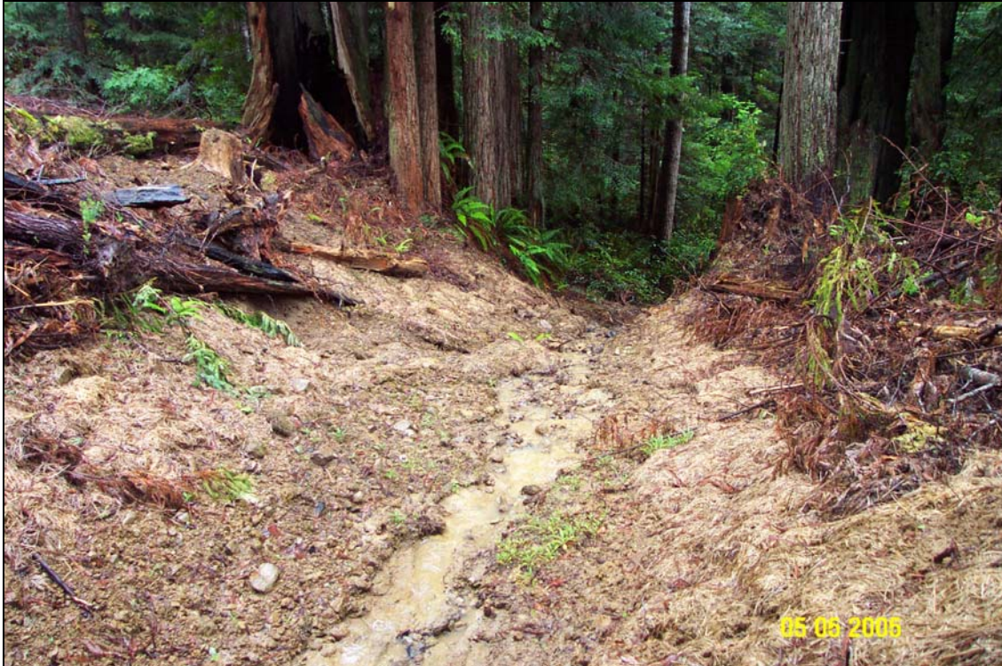
Photo 4. Stream crossing Site #18 approximately one year after decommissioning. Picture was taken from above the right side slope near the upper end of the excavation looking toward the bot.
