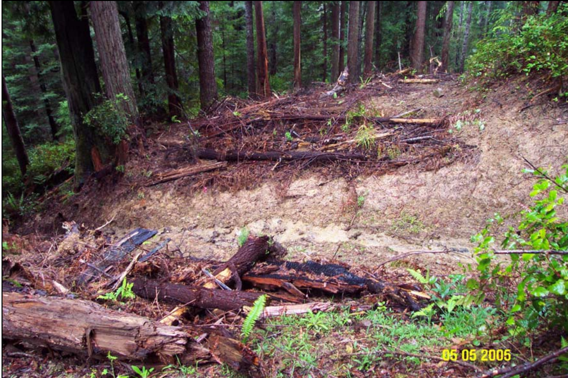
Photo 3. Stream crossing Site #18 approximately one year after decommissioning. Picture was taken from above the left side slope near the upper end of the excavation with the downstream end of the excavation (the bot) on the left side of the photo.
