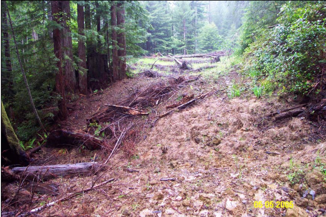
Photo #20. Site #8 almost one year after treatment. View is similar to the photo above. A swale was excavated to direct spring flow toward the lower end of site #8, and is located just beyond the slash pile in the center of the photo.
