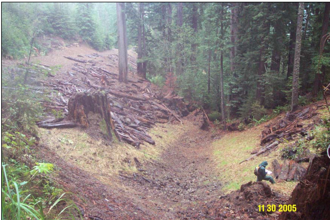
Photos 11A and 11B. R14 Road, site #145.2, pre and post treatment. View is from the top of the excavation. Note the slash and woody debris generated at the site are placed upon the freshly excavated surfaces. Note the person, located in the lower right corner of the bottom photo, for scale. Site #145.1 was located on the left road approach to this site.
