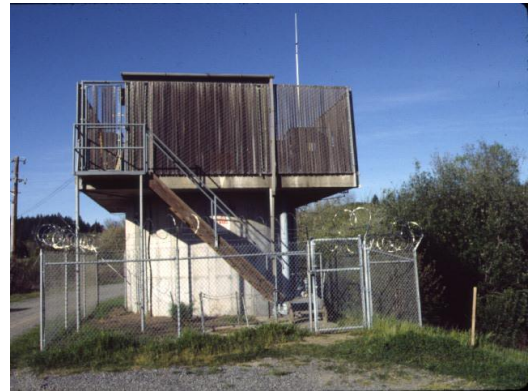
The early warning system "alpha site" at the Wohler Dam Ranney collector. River water was pumped from below the dam to the right of the photo.
