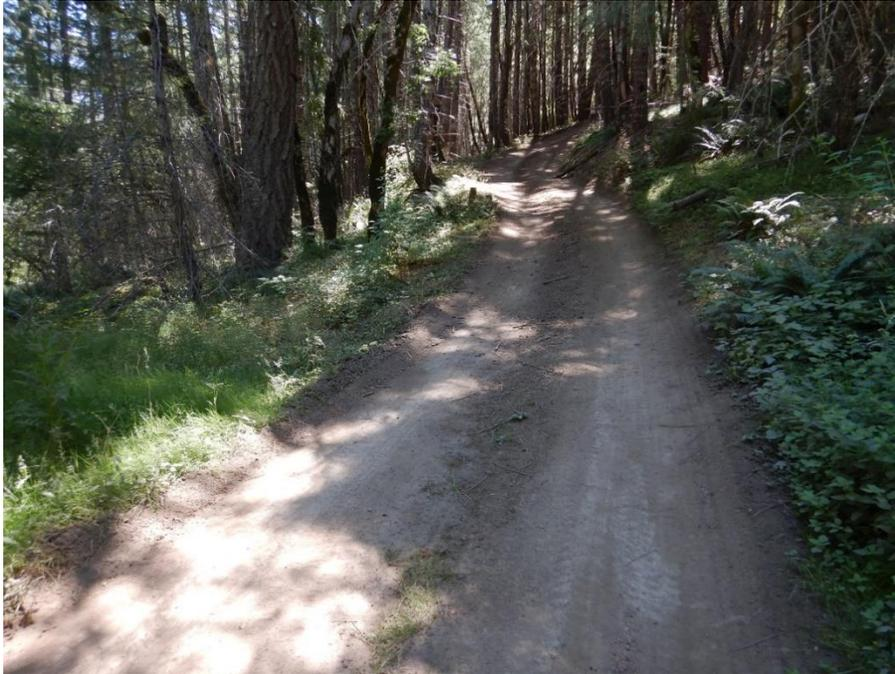
*Figure 2— Looking east along a dirt road approaching a stream crossing on the Szagora LLC property. The road is steep and lacks key features, such as water bars or rolling dips, to direct stormwater off the road and minimize sediment delivery to the stream. This leaves the road's earthen surface susceptible to erosion by stormwater, which is likely to carry excess fine sediment from the road into the stream.*
