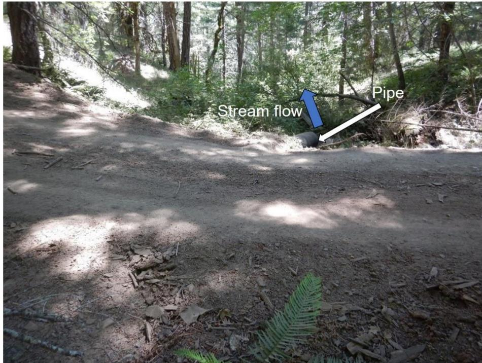
*Figure 1—Photo looking downstream at the road crossing an unnamed tributary to the Mad River on the Szagora LLC property. The existing culvert is too small and does not meet industry sizing standards. Thus, when the stream is running full, water can flood the road and carry road material and fine sediment back into the waterways. Fine sediment can make it difficult for fish to breathe, find food and refuge, and reproduce.*
