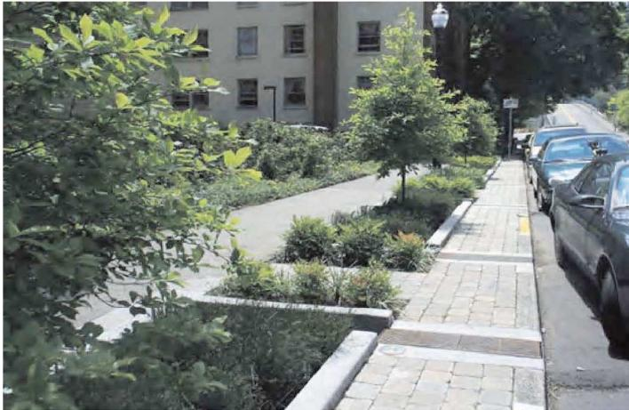
Figure 7: Flow-through planter (*Model for Living Streets Design Manual, 2011*).
