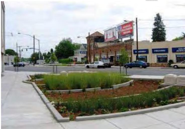
Figure 2: Bioretention system (*Model for Living Streets Design Manual, 2011*).
