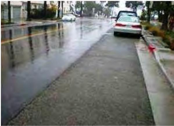
Figure 5: Permeable pavement during a storm event (*Model for Living Streets Design Manual, 2011*).
