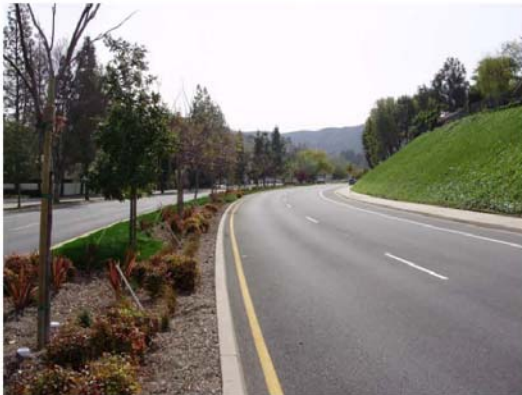
Figure 2: After Photo showing bio-swale eliminating runoff and providing pollutant mitigation via infiltration.
