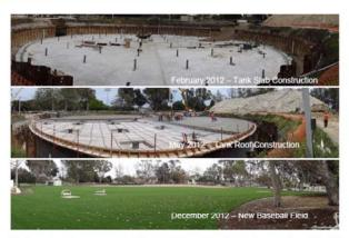
The dry weather storm water run off and first flush flow during the rain events is diverted into the detention tank at 11,000 gallon per minute for 4 hours where it is held for 72 hours prior to discharge into the sewer system.
