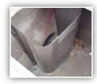
and prevent trash from entering the City storm drain system. Each CB opening screen cover has a self-opening device activated by a predetermined street gutter flow to disengage its locking mechanism. The CB inserts are perforated screens that are installed inside the CB in front of the outlet pipe of the catch basin.
