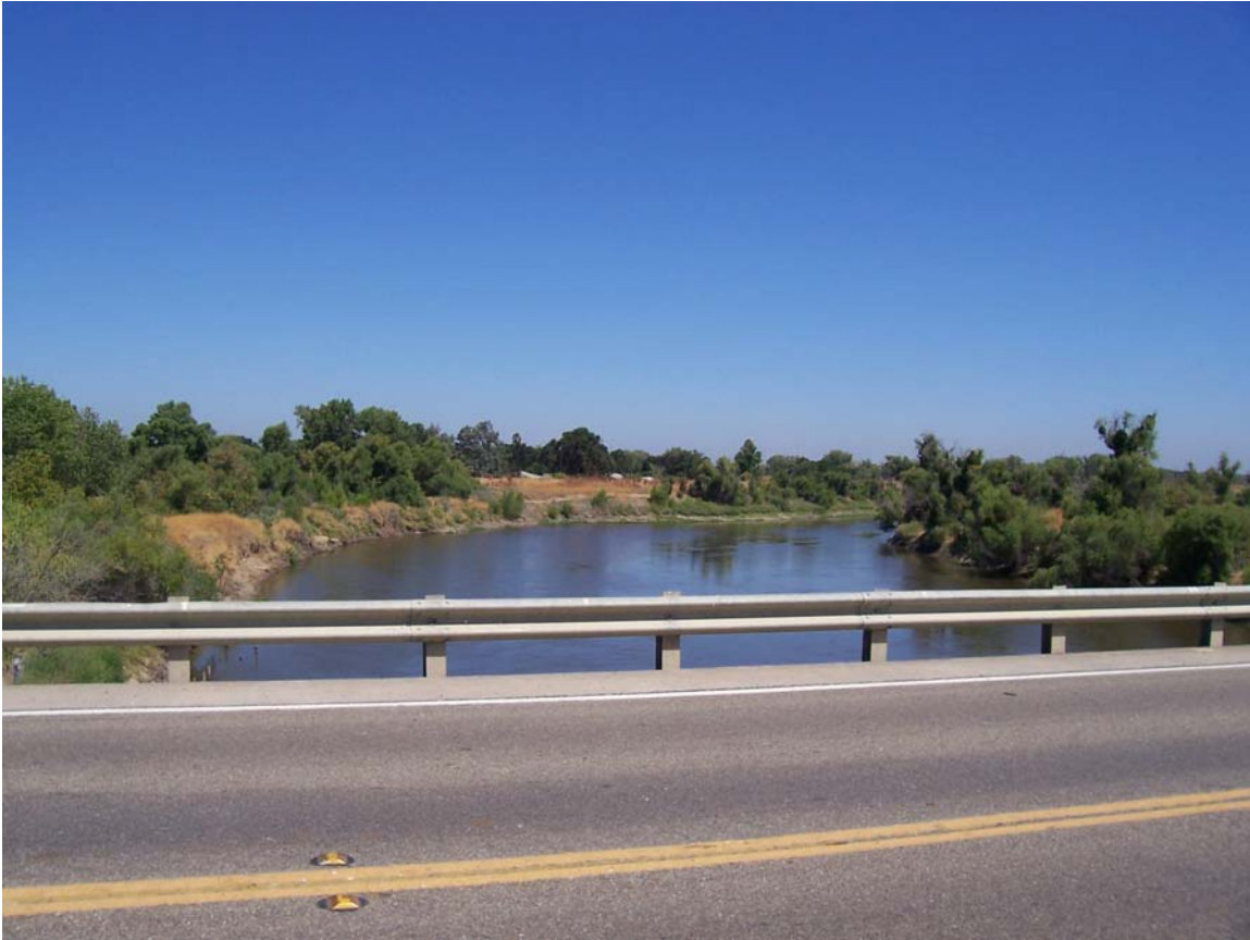
SJR @ Airport Way, 07-22-2010, Facing North (downstream)
