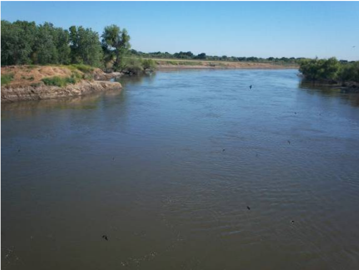
SJR @ Maze Blvd, 05-10-2011, Facing North (downstream)
