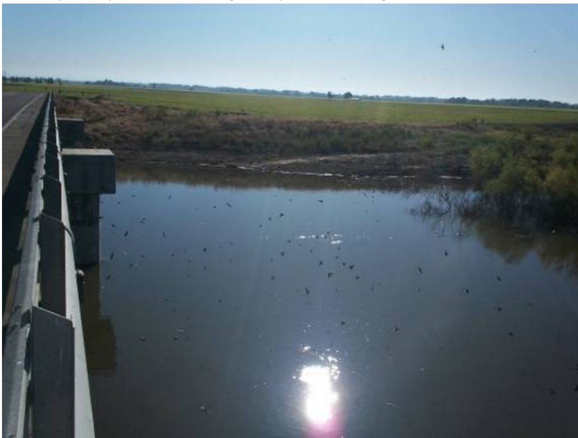
SJR @ Airport Way, 05-10-2011, Facing East (upstream to the right)
