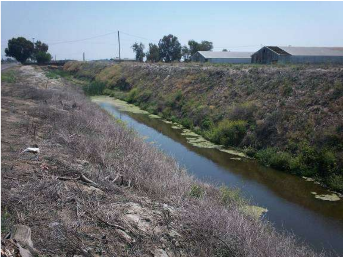
Levee Drain @ Carpenter Rd, 05-09-2012, Facing South (downstream)
