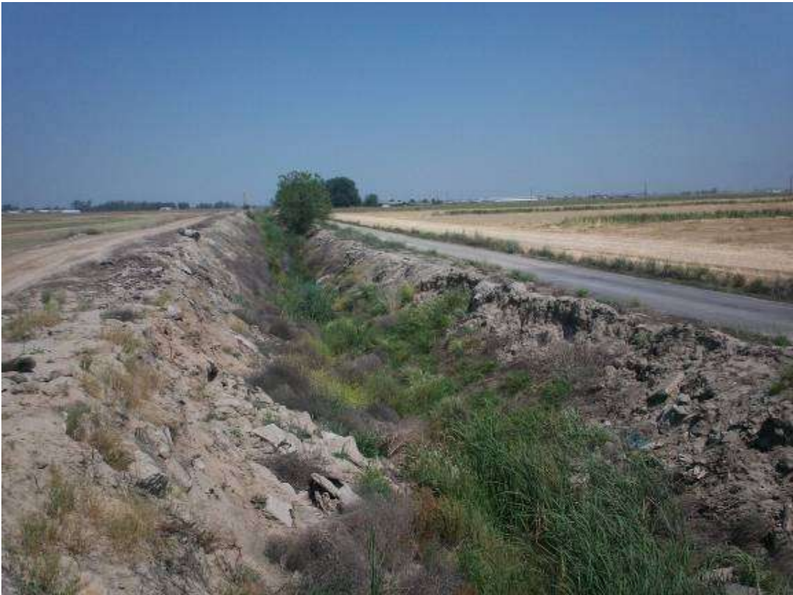
Levee Drain @ Carpenter Rd, 05-09-2012, Facing East (upstream)
