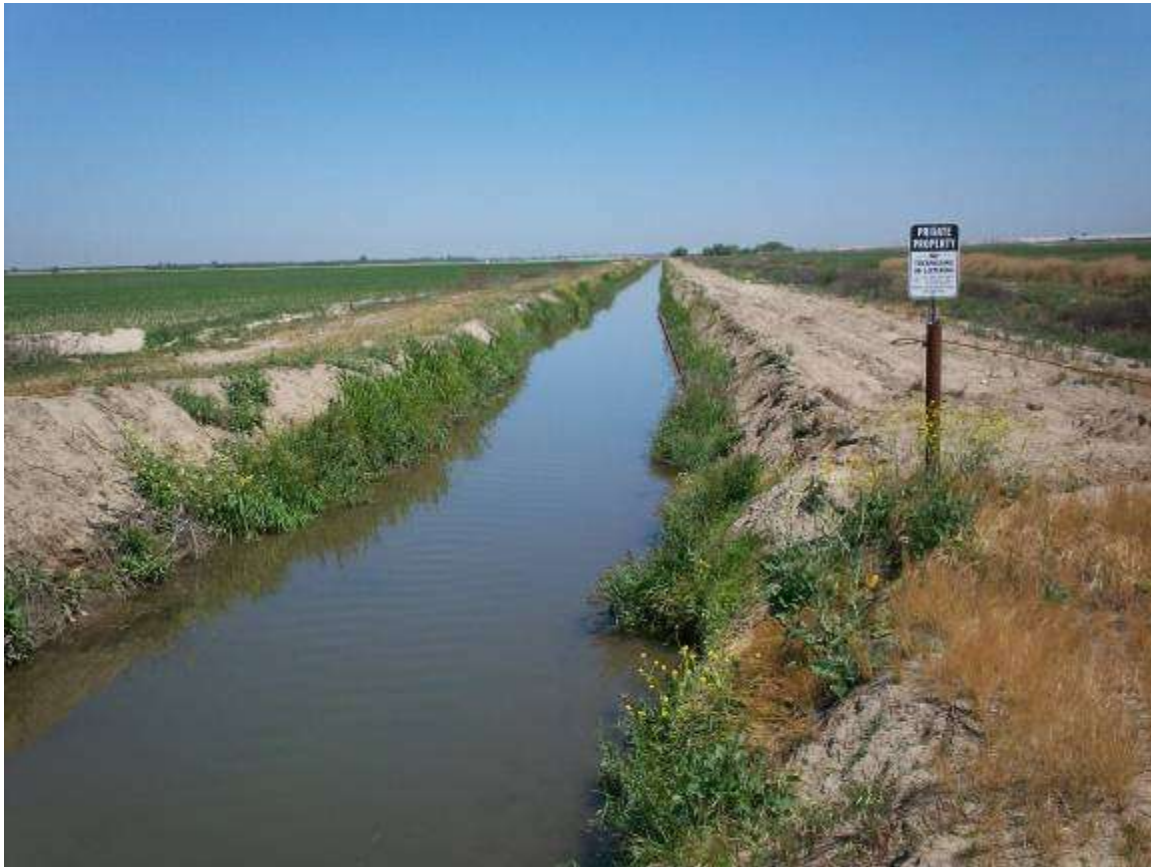
McCoy Lateral @ Hwy 140, 05-09-2012, Facing North (upstream)
