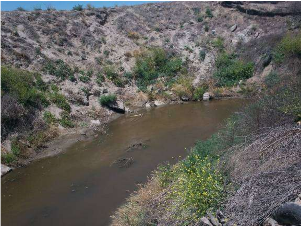
Levee Drain @ Carpenter Rd, 06-12-2012, Facing North (upstream)
