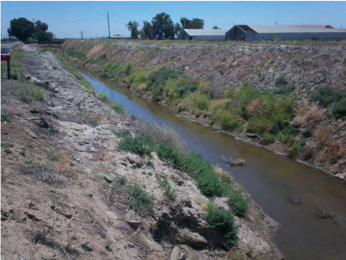
Levee Drain @ Carpenter Rd, 06-12-2012, Facing South (downstream)
