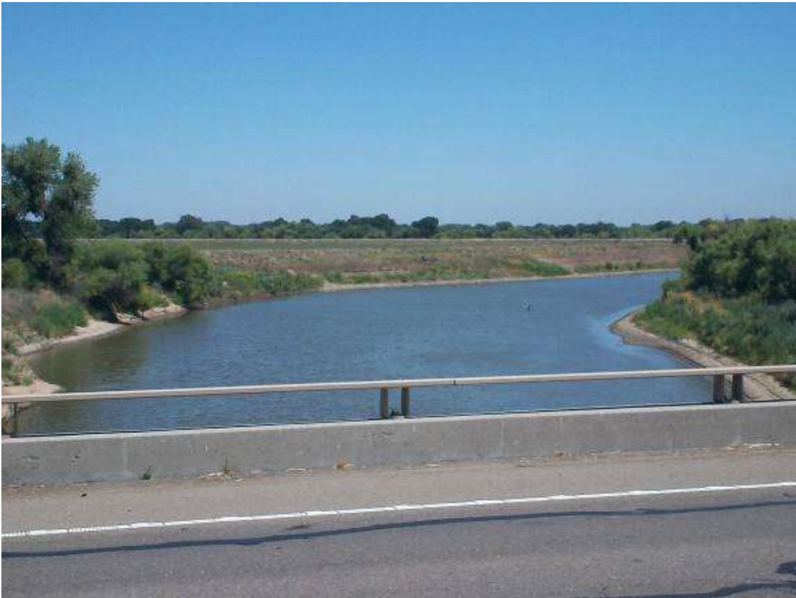
SJR @ Maze Blvd, 06-12-2012, Facing North (downstream)
