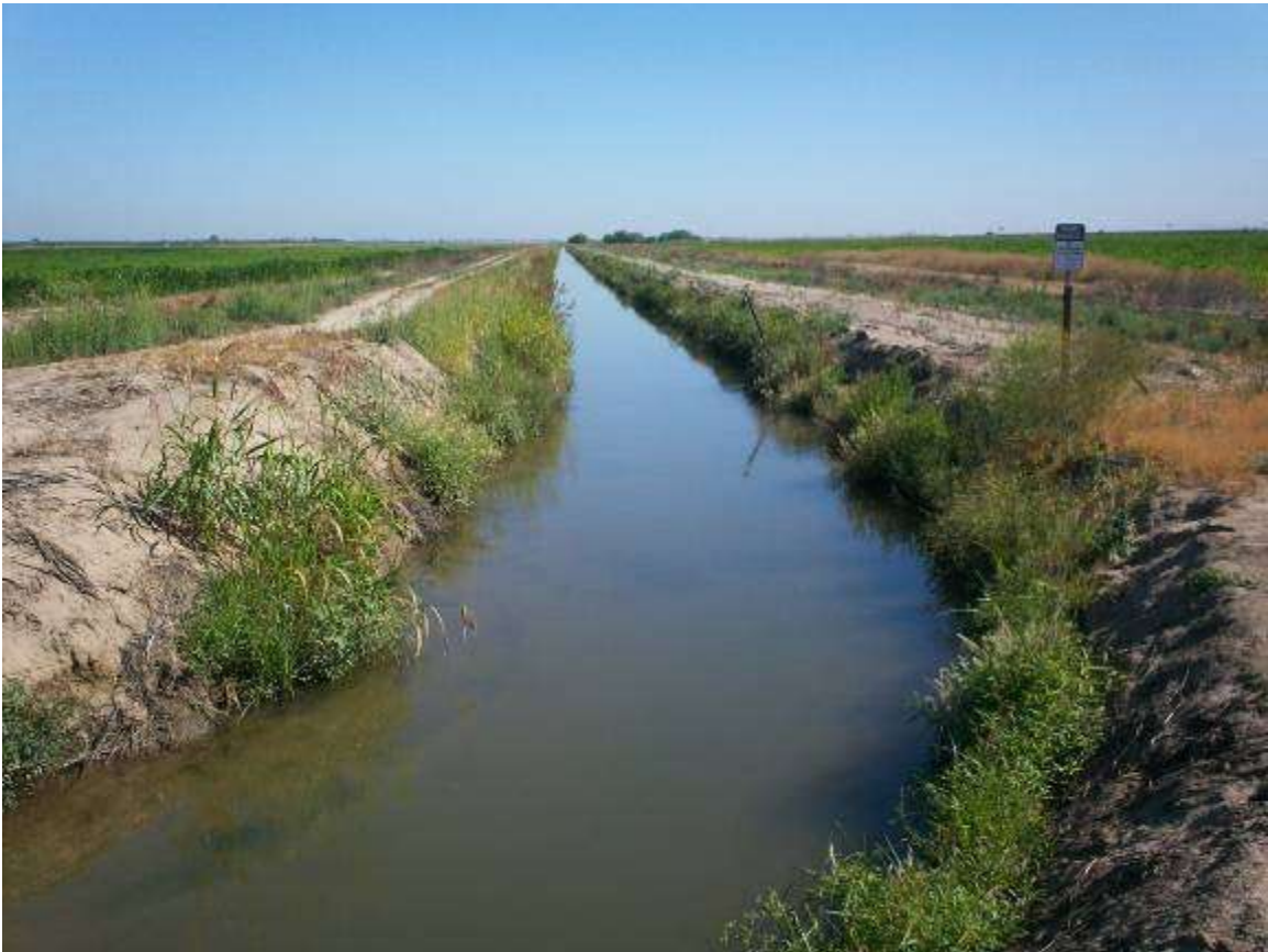
McCoy Lateral @ Hwy 140, 06-12-2012, Facing North (upstream)
