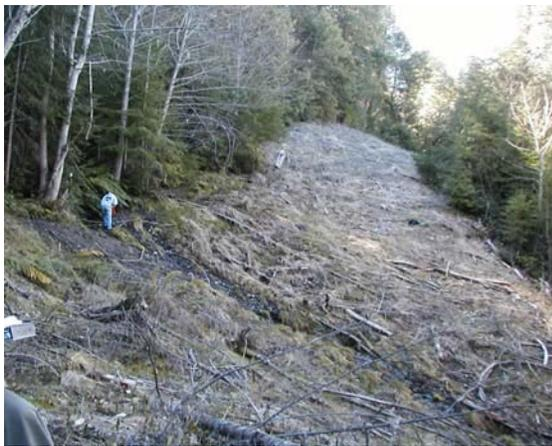
Photo 7 shows a typical untreated roadbed left between restored stream crossings. Photo 8 is an example of road prism outsloping where slope stability was a concern.
