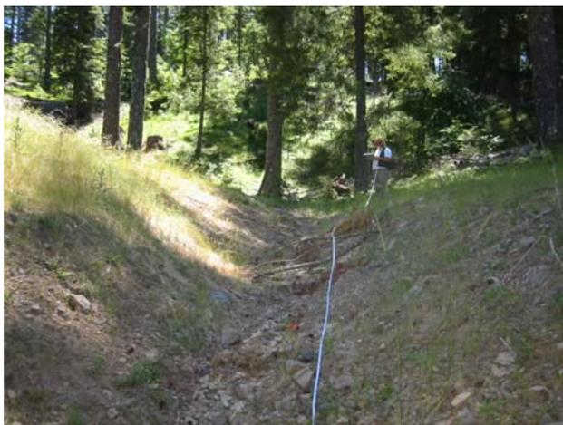
Restoration of stream crossings must be carefully planned and executed, but even the best-designed projects have some post-treatment channel erosion. Some of these erosional features can be avoided while others are unpredictable and probably unavoidable. During site excavation, unforeseen
