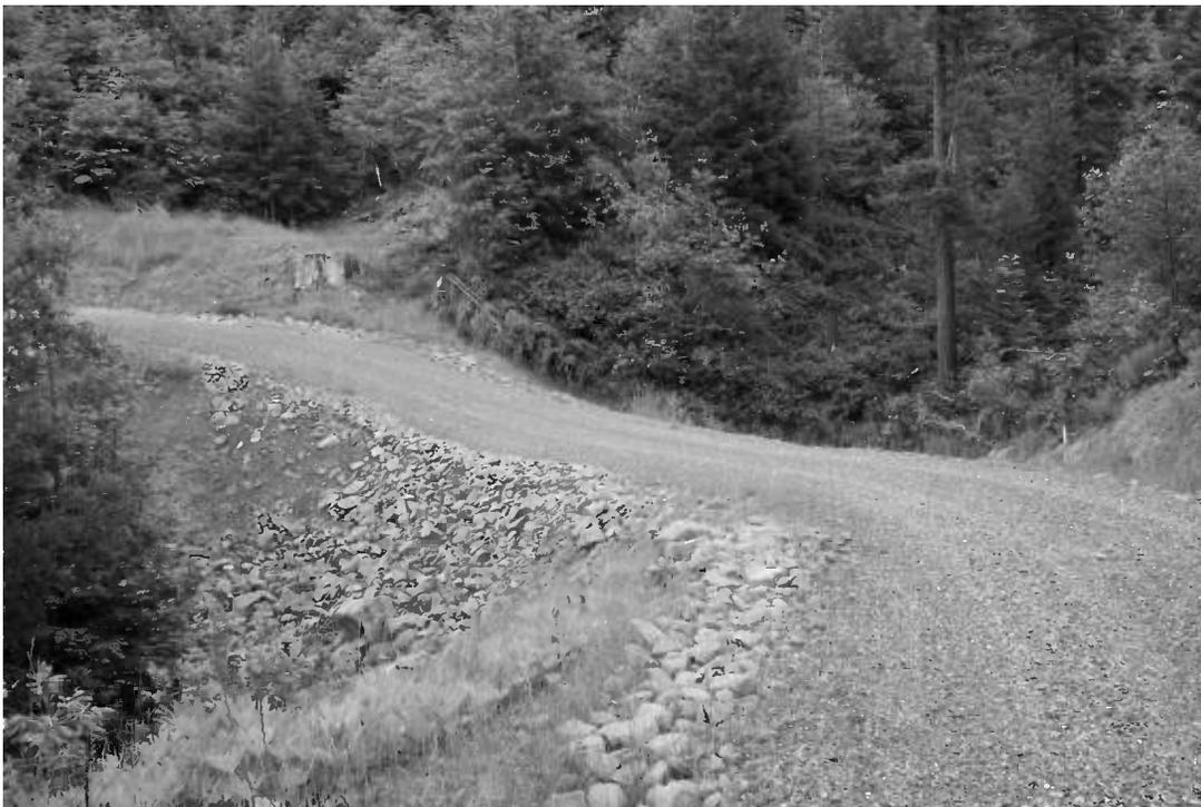
Figure 7. Typical crossing and road installation, PALCO lands, Humboldt County. Design features include alignment and slope of culvert conforming to the natural channel, extensive armoring to prevent fill slope and channel erosion, and provision of a "critical dip" in the road surface to prevent diversion of flow down the road if the culvert plugs. All exposed soils were treated with straw mulch and grass seeding to prevent erosion.
