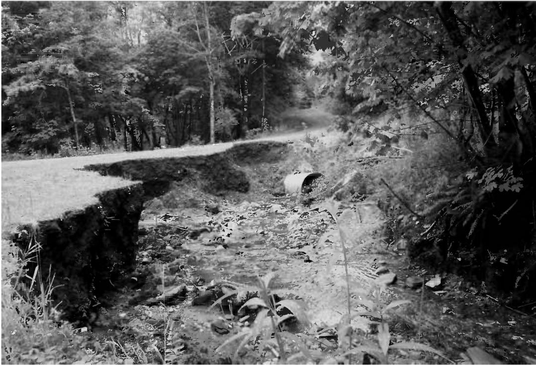
Figure 6. Erosion of road fill at site 19 at Hoopa caused by temporary culvert plugging from landslide debris and sediment. Incision occurred downstream as well.
