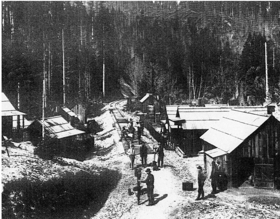
Figure 3. A) Work crews collect blasted hillslope material just east of the Bunker Gulch tunnel. This material was used to construct the railroad grade into the SFNR basin. Photo dated approximately 1904 (Wurm, 1986). B) The railroad reaches Camp 1 at the confluence of the SFNR and North Fork Of the SFNR. The town is built on a large pre-historic terrace and served as the woods headquarters of the Caspar Lumber Company. Photo dated approximately 1904 (Wurm, 1986).
