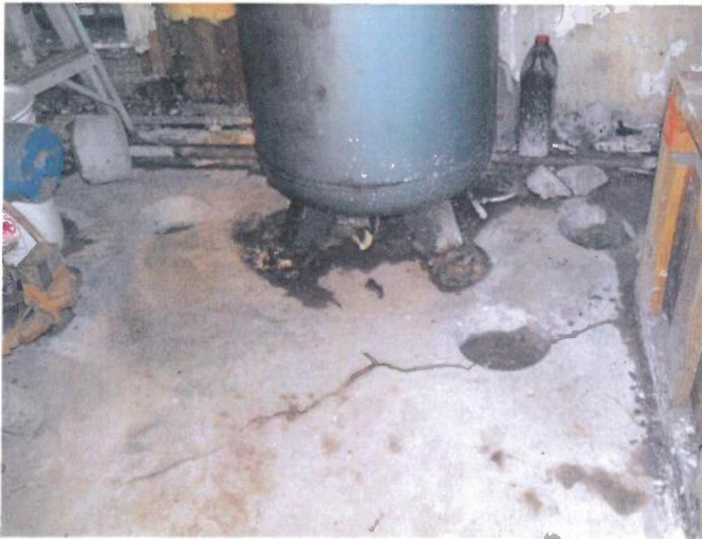
**Photo 1:** View of three soil borings in boiler room. B-A on left, B-B on upper right, and B-C on lower right side of photo. Floor crack at B-C readily visible on left side of photo.
