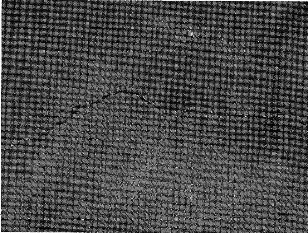
**Photo 7:** View of crack following 5-gallon pour test. Note width of crack and lack of pooled water. Also, some small white flecks are visible in crack, having got caught as water fell into crack.
