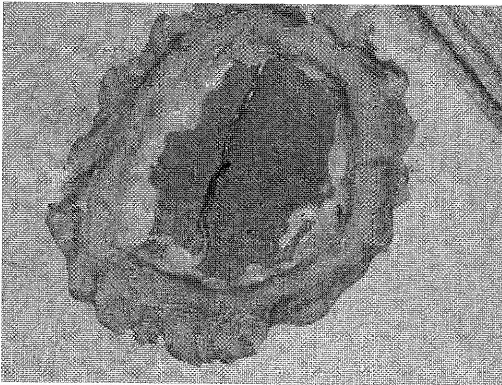
**Photo 4:** Close-up view of pour test in clay basin, just southwest of sink/drain area. Again, open crack, where water fell through crack, is visible on lower side of photo.
