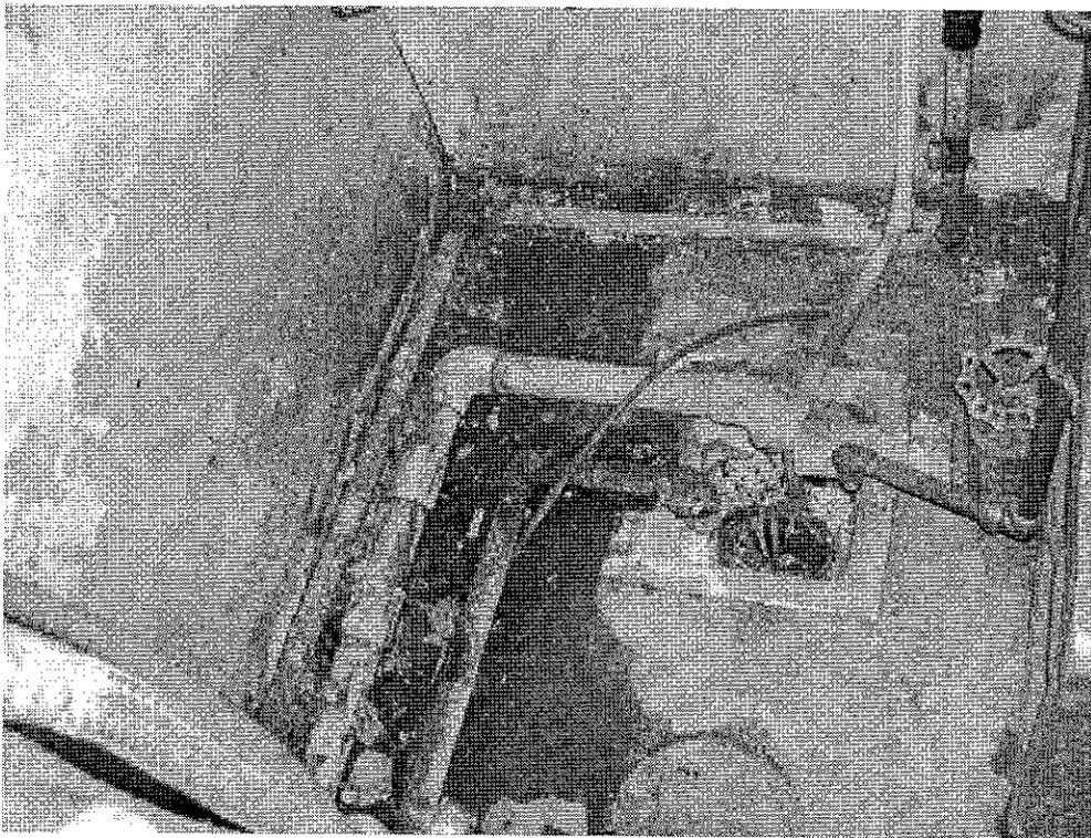
**Photo 2:** View of floor sink/drain area. Note crack in concrete on lower right side of photo, emanating from corner of sink. Boiler water collects along left wall because there are no breaches in concrete at that location (crack area is normally dry).
