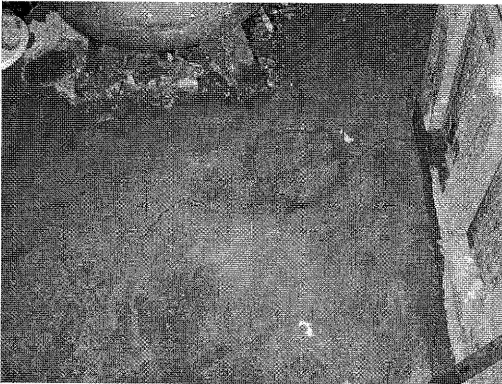
**Photo 6:** View of crack following 5-gallon pour test. Note width of crack and lack of pooled water. Also, some small white flecks are visible in crack, having got caught as water fell into crack.
