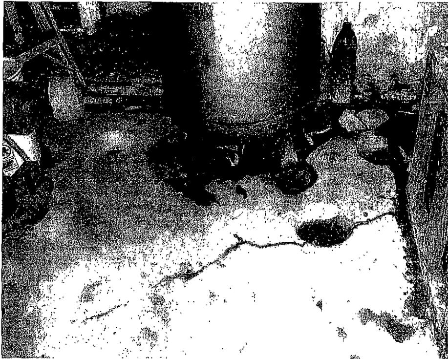
**Photo 1:** View of three soil borings in boiler room. B-A on left, B-B on upper right, and B-C on lower right side of photo. Floor crack at B-C readily visible on left side of photo.
