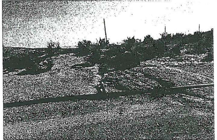
Photograph 8. – View of hose west of tankfarm.
