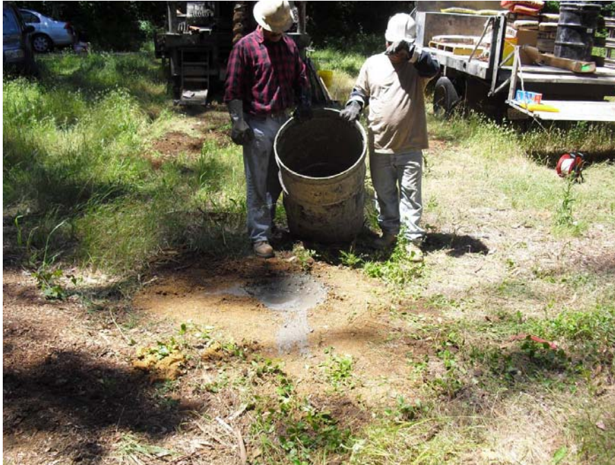
Backfilling Adobe Gulch boring AG-SM-1
