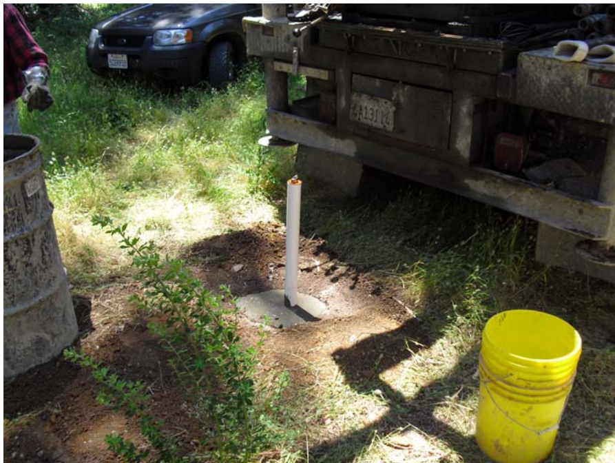
Completion of Adobe Gulch piezometer AG-PM-1
