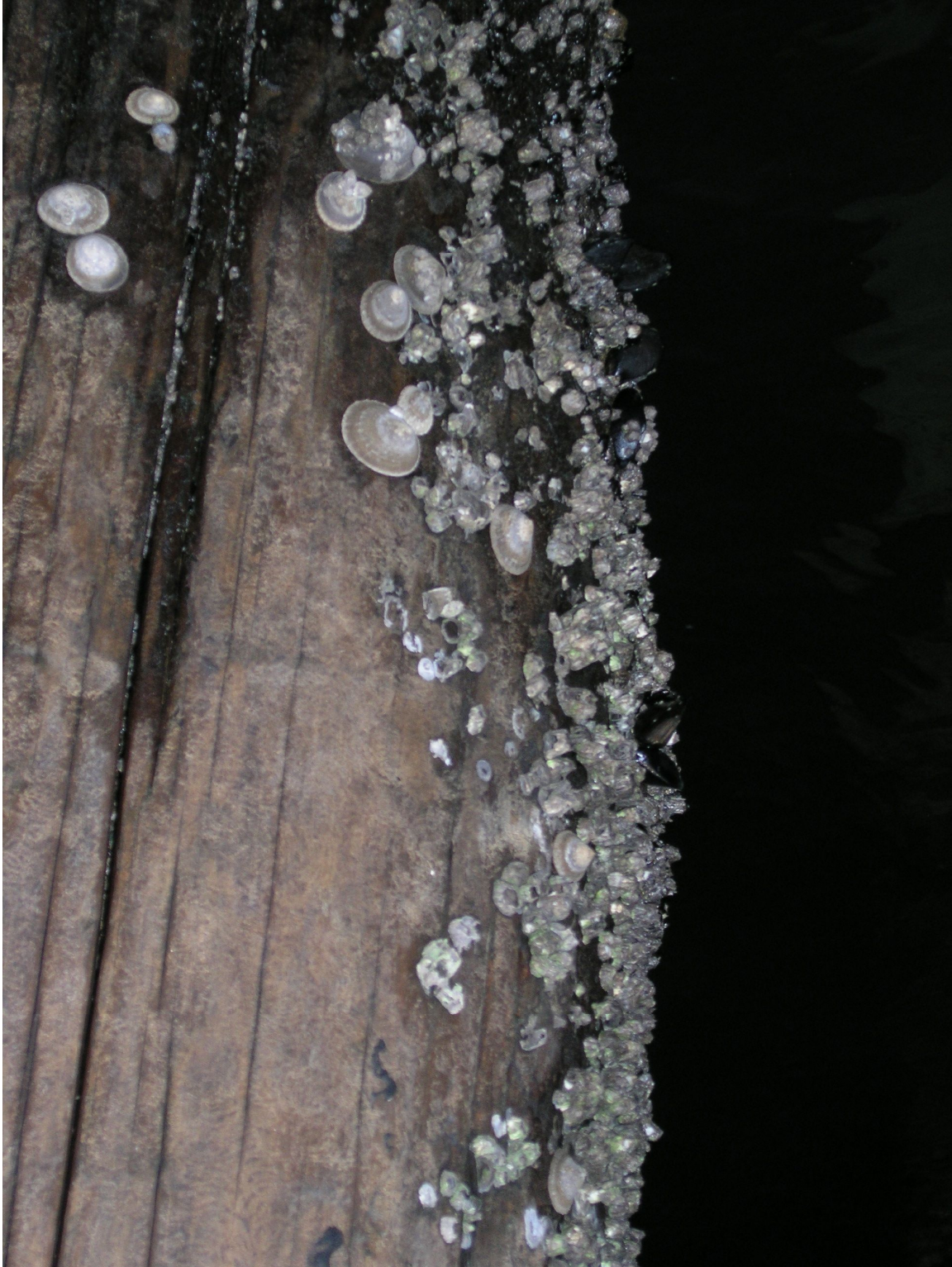
Figure 4. Barnacles dominate the pilings in the high intertidal zone at the site; native oysters, mussels and limpets are also present.
