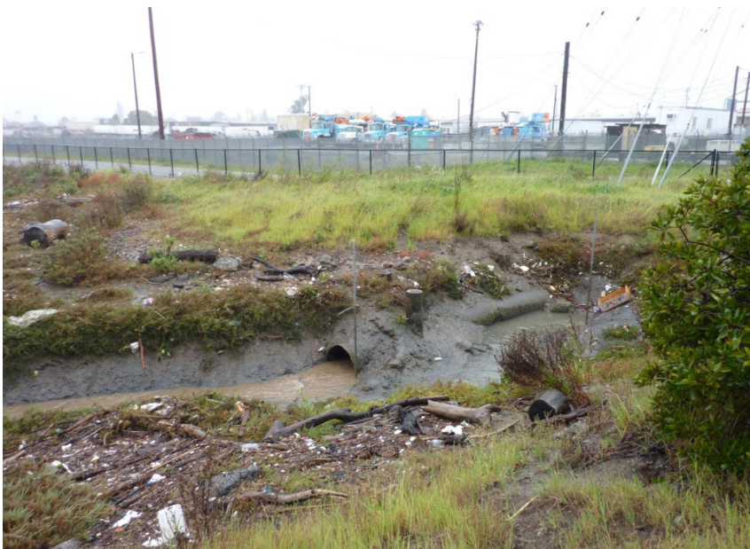
Figure 2. Northwest-facing view of a storm drain near East Creek Slough in the Martin Luther King Jr. Regional Shoreline, Oakland. Photo taken by Ian Wren on March 14, 2012
