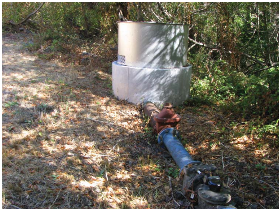
Photograph 5: Town of Hillsborough's water pipe connected to SFPUC water system (9-18-2015 HTK)
