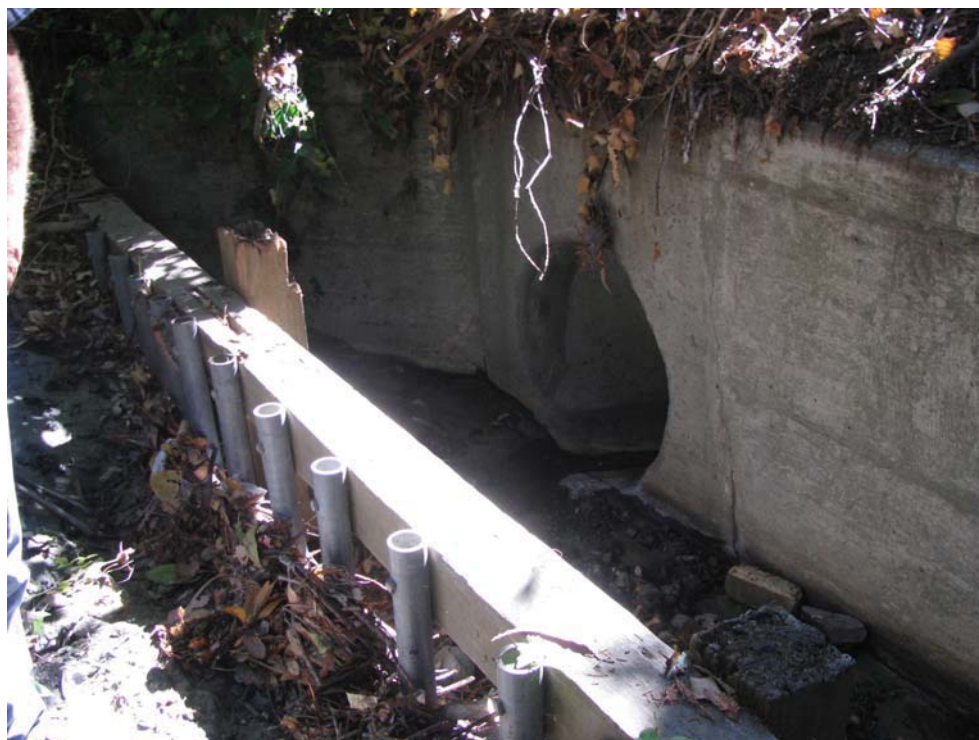
Photograph 14: Trash and woody debris interceptor and an inlet of about 3,100 feet long concrete drainage pipe that daylights at San Mateo Creek (9-18-2015 HTK)
