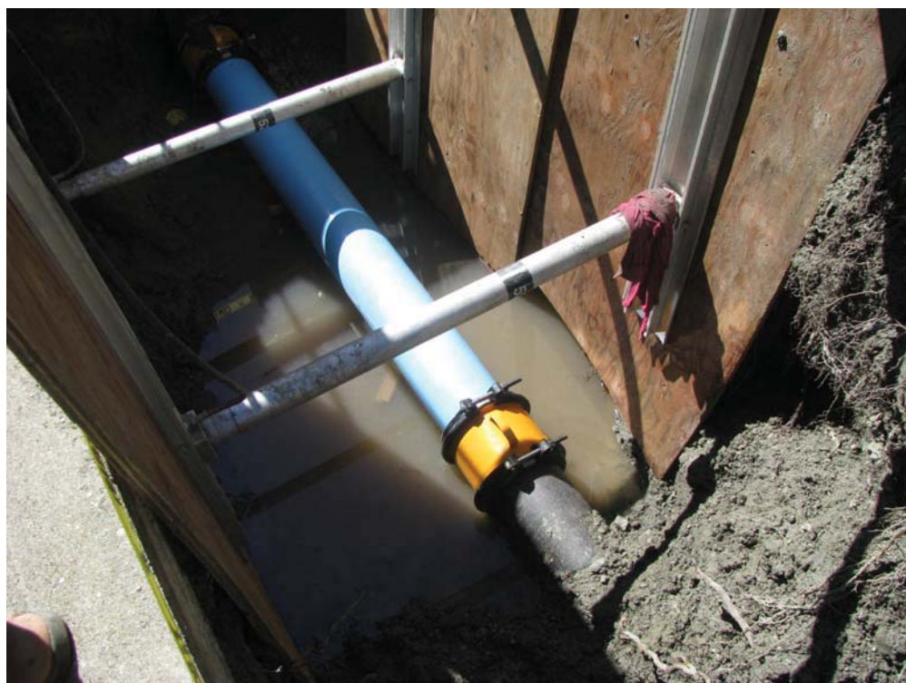
Photograph 10: Excavated discharge location showing a repaired 8-inch water main pipe about 6 feet below grade (9-18-2015 HTK)
