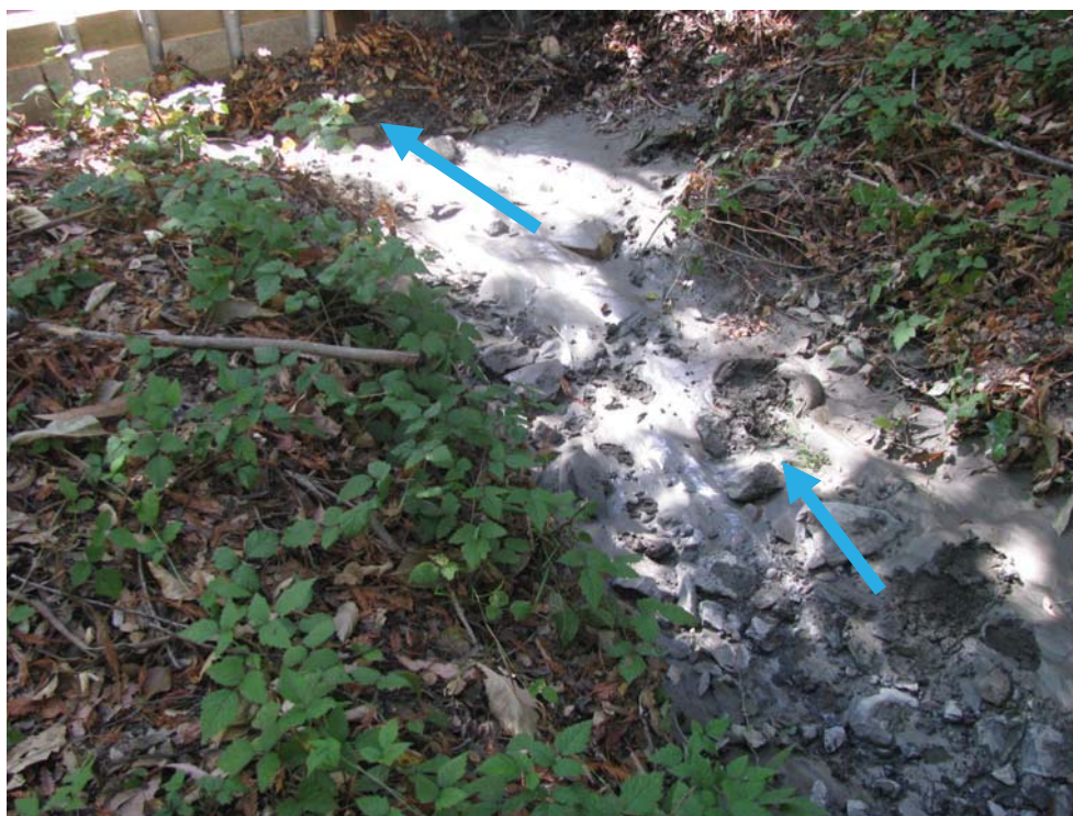
Photograph 13: Sediment deposition behind a trash and woody debris interceptor along the unnamed open drainage (9-18-2015 HTK)
