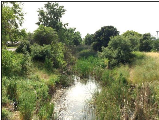
Photo 6-1: The maintained reach of Sheehy Creek looking downstream from the Kelly Road culvert, showing channel roughness.
