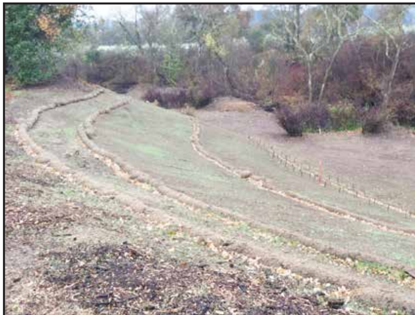
COIR LOG INSTALLATION (TYP) - SECTION VIEW
