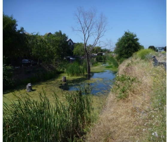
Photo 3-2: The downstream portion of Tulucay Creek Reach 1 looking downstream showing channel roughness and inundation from beaver activity. n=0.04-0.05
