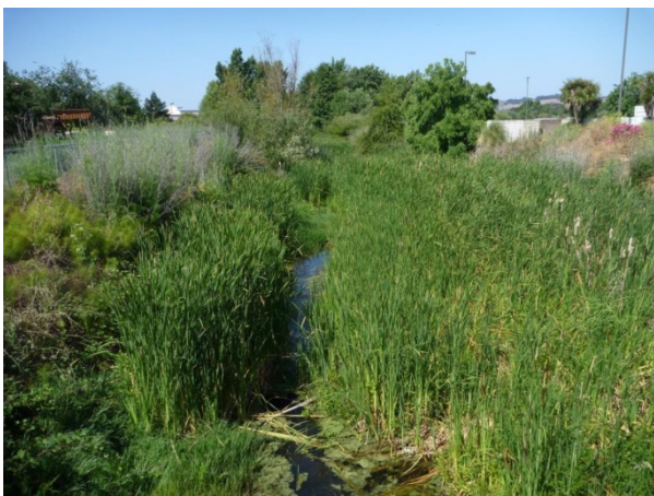
Photo 3-3: Tulucay Creek Reach 2 looking downstream from Soscol Avenue bridge showing channel roughness. n=0.1-0.15
