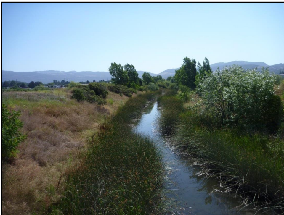
Figure 8. Tulucay Creek Reach 2 looking upstream from the railroad bridge at the downstream boundary of the reach, showing channel roughness. n=0.04-0.045
