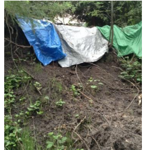
Photo 23: Erosion along bank due to fallen tree, repair
