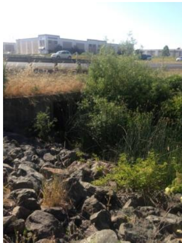
Photo 25: Vegetation blocking downstream box culvert on Sheehy Creek
