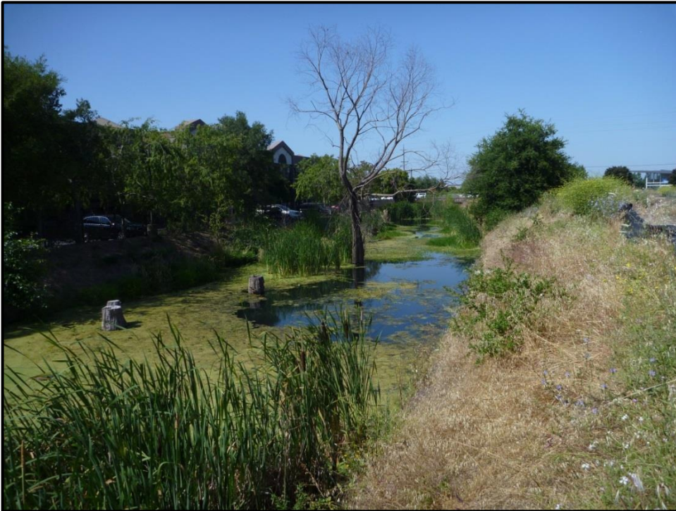
Figure 6. The downstream portion of Tulucay Creek Reach 1 looking downstream showing channel roughness and inundation from beaver activity. n=0.04-0.05
