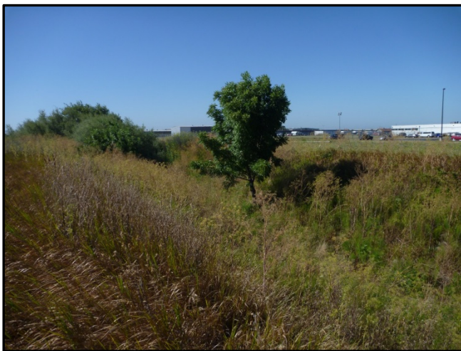
Photo 5-1: The upstream portion of the Fagan Creek maintenance reach, looking obliquely upstream from the right bank, showing channel roughness.
