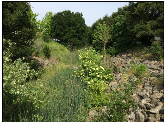
Photo 6-2: The maintained reach of Sheehy Creek looking upstream from the Hwy 29 culvert, showing channel roughness.
