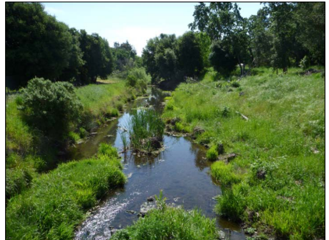
Photo 2-4: Reach 2 looking downstream showing channel roughness. n=0.030-0.040
