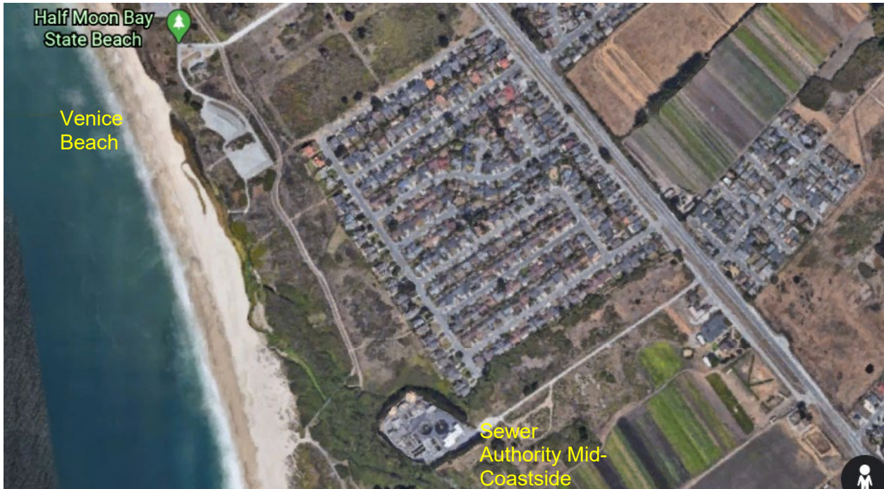
Figure 4-5 Municipal Sewage Treatment Plant in Half Moon Bay
