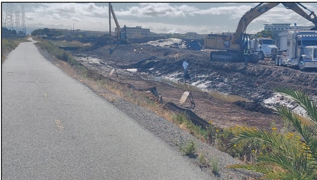
Figure 5: Offsite Ditch Sediment Remediation in Progress
