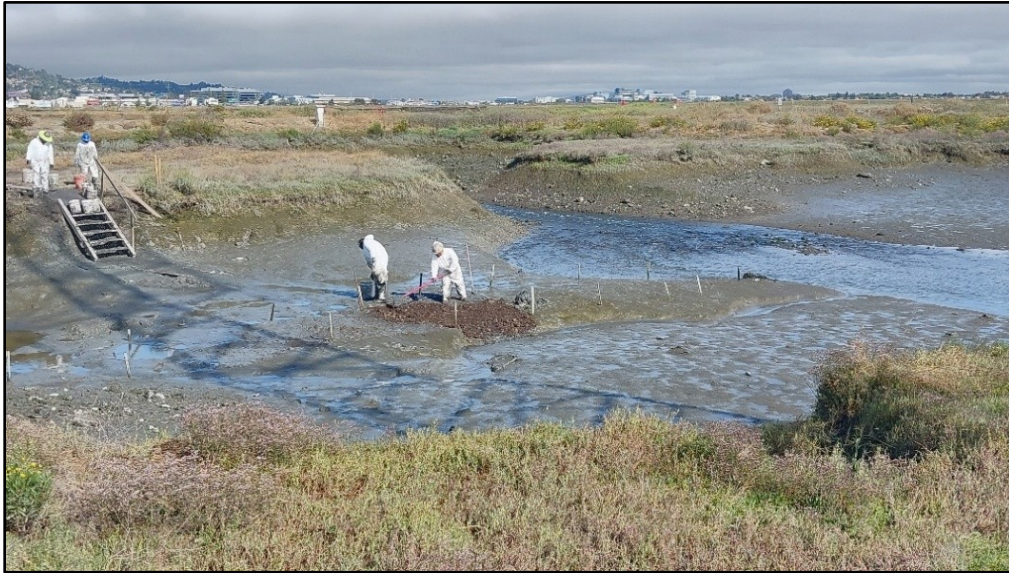
Figure 4: Sediment Cleanup Using Hand Tools, Smith Slough
