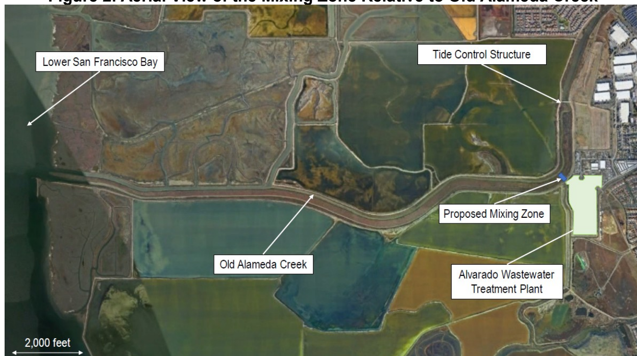
Figure 2. Aerial View of the Mixing Zone Relative to Old Alameda Creek
