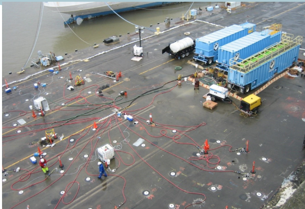
Photo below: Remedial injections at Mare Island
