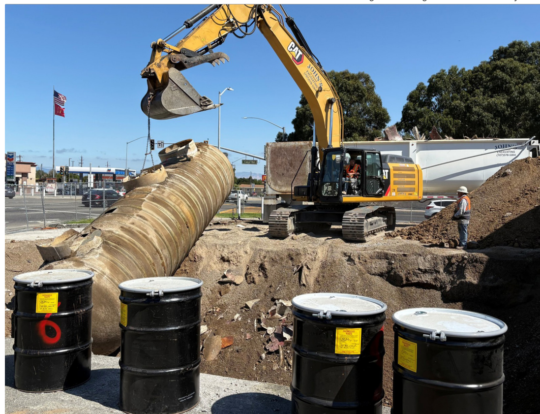
Photo below: Underground storage tank excavation, Bay Point
