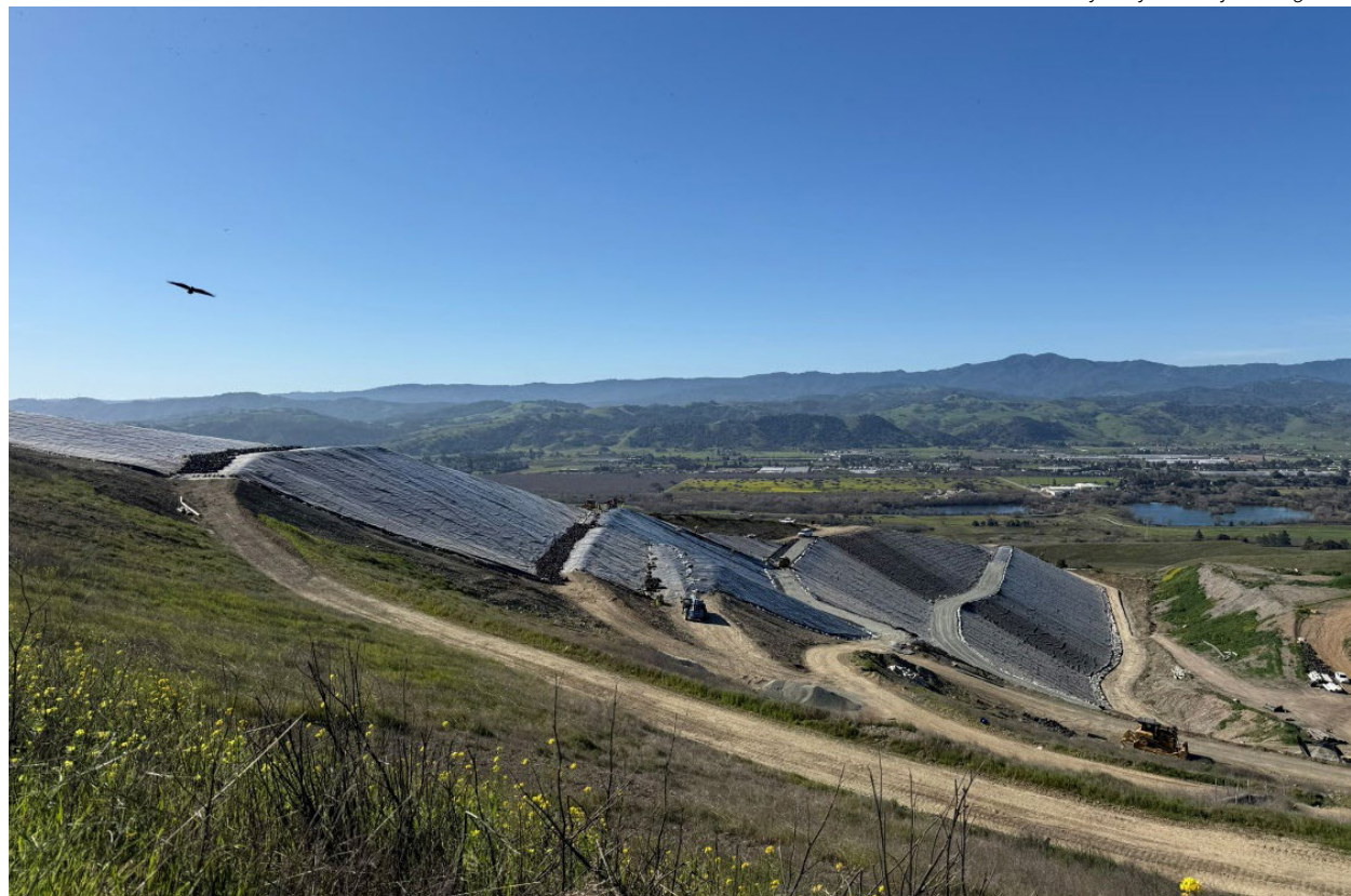
Photo below: Kirby Canyon Landfill, Morgan Hill
