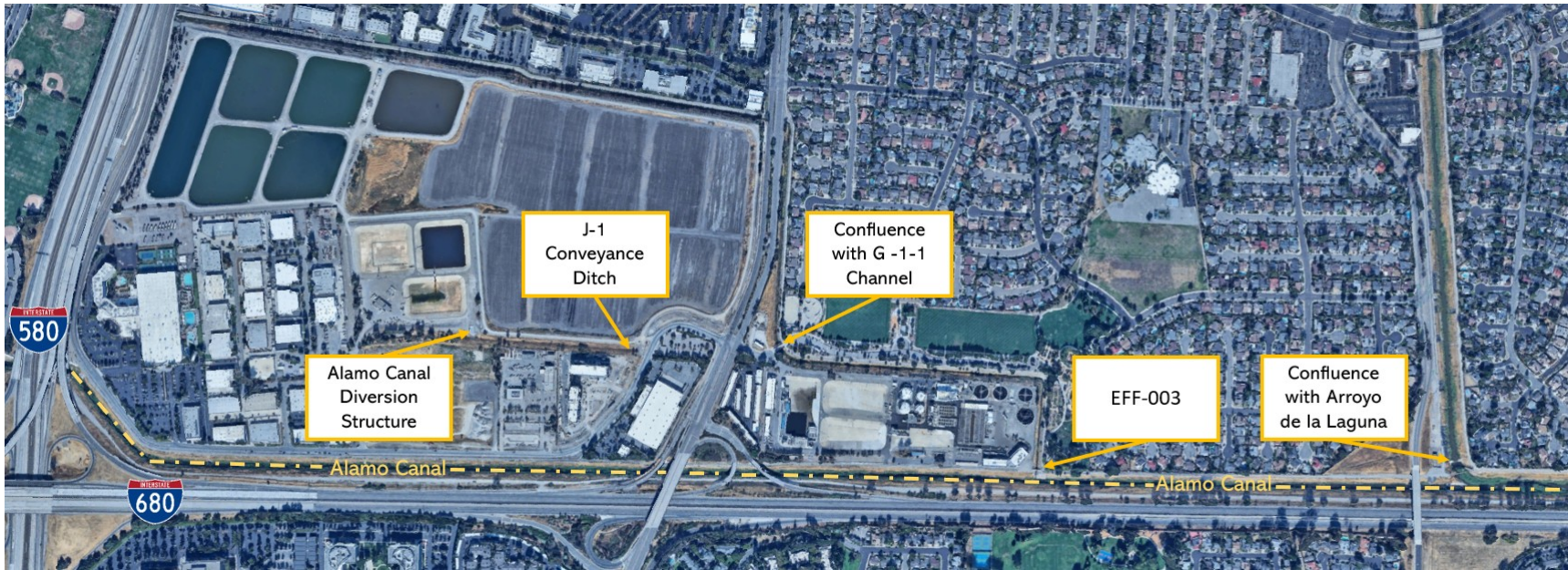
Figure B-3. Aerial View of Alamo Canal Outfall and Surroundings
