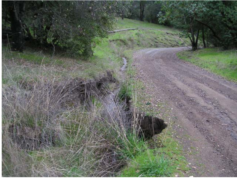
Figure 4. Rills and Gullies on a Compacted Dirt Road Gully forms where runoff depth and slope are sufficient to erode soft colluvium at this site, which is underlain by the mélange bedrock unit.
