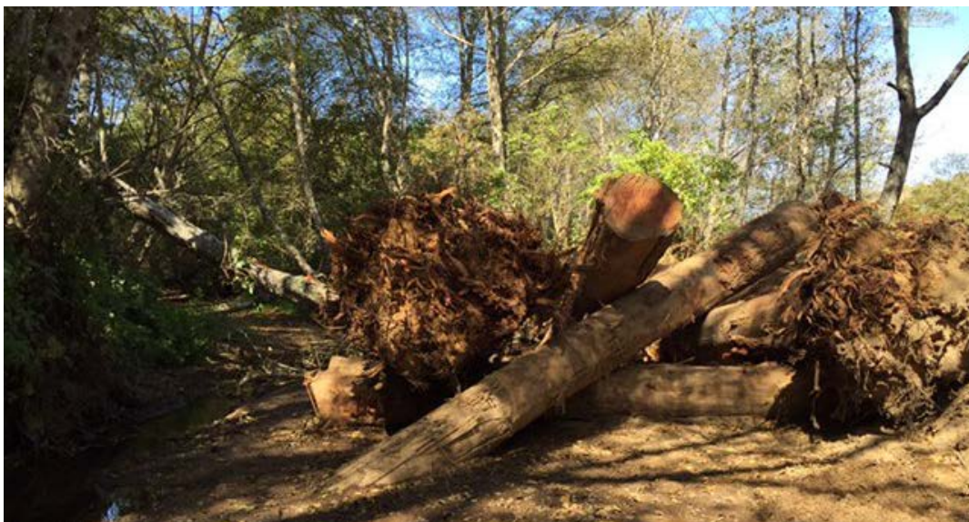
Figure 44. A large wood structure constructed for the Butano Farms floodplain restoration project
