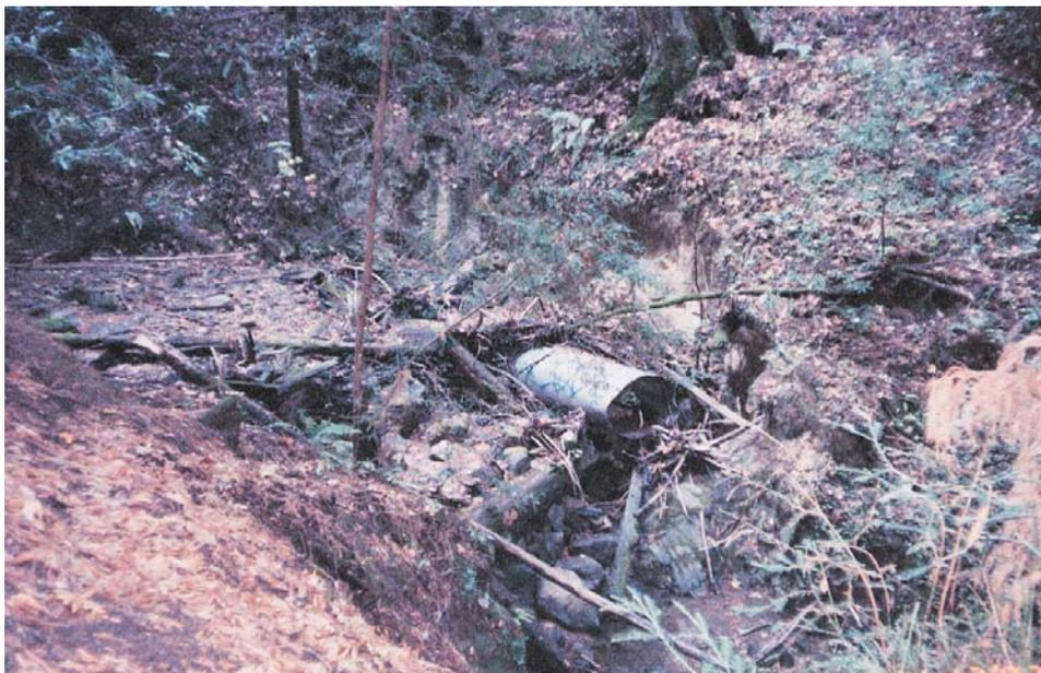
Site 15      Martin Creek about 200 ft upstream of Old La Honda Road crossing, looking upstream at erosion of unpaved road crossing
