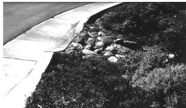
**Inlet detail for urban curb/swale system**
