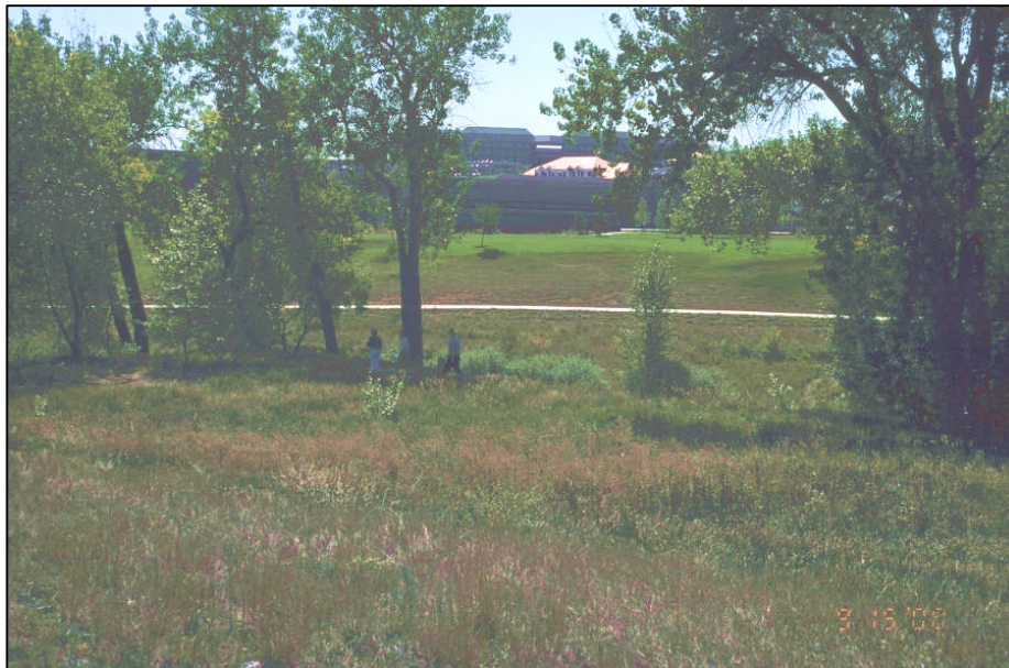
Photograph MD-5—Natural channel (open floodplain design) serving as a major drainageway. Note the preservation of riparian vegetation, absence of floodplain encroachment and the use of grade control structures to arrest thalweg downcutting (i.e., channel incising/degradation)
