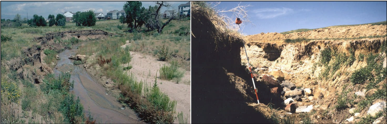
Photograph MD-4—Channel degradation in an unstable channel.
