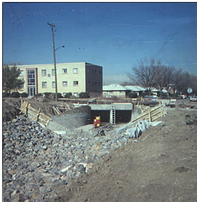
Photograph MD-9—Riprap channel. Burying and revegetation of the rock (i.e., soil riprap) could make this site blend into the adjacent terrain very nicely.
