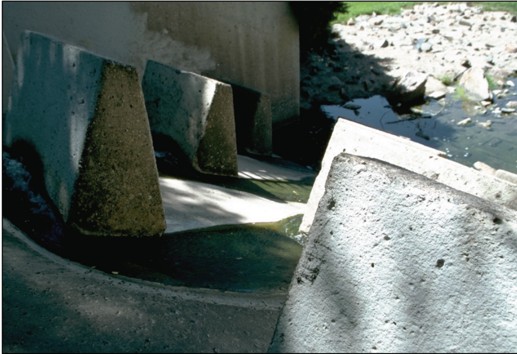
Photograph HS-9—Close-up of the inside workings of a baffle chute drop after more than three decades of service.
