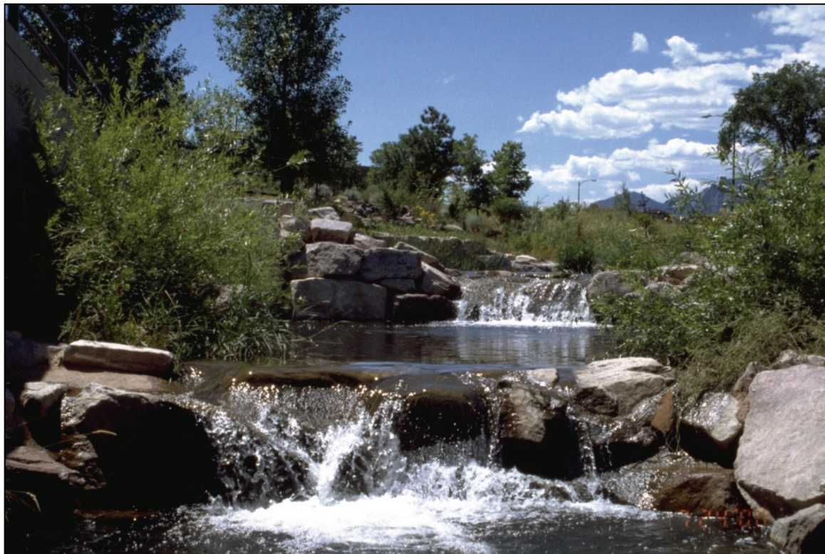
Photograph HS-17—Grouted sloping boulder drops can be built in series to create pleasing amenities and to provide stable and long-lived grade control structures.
