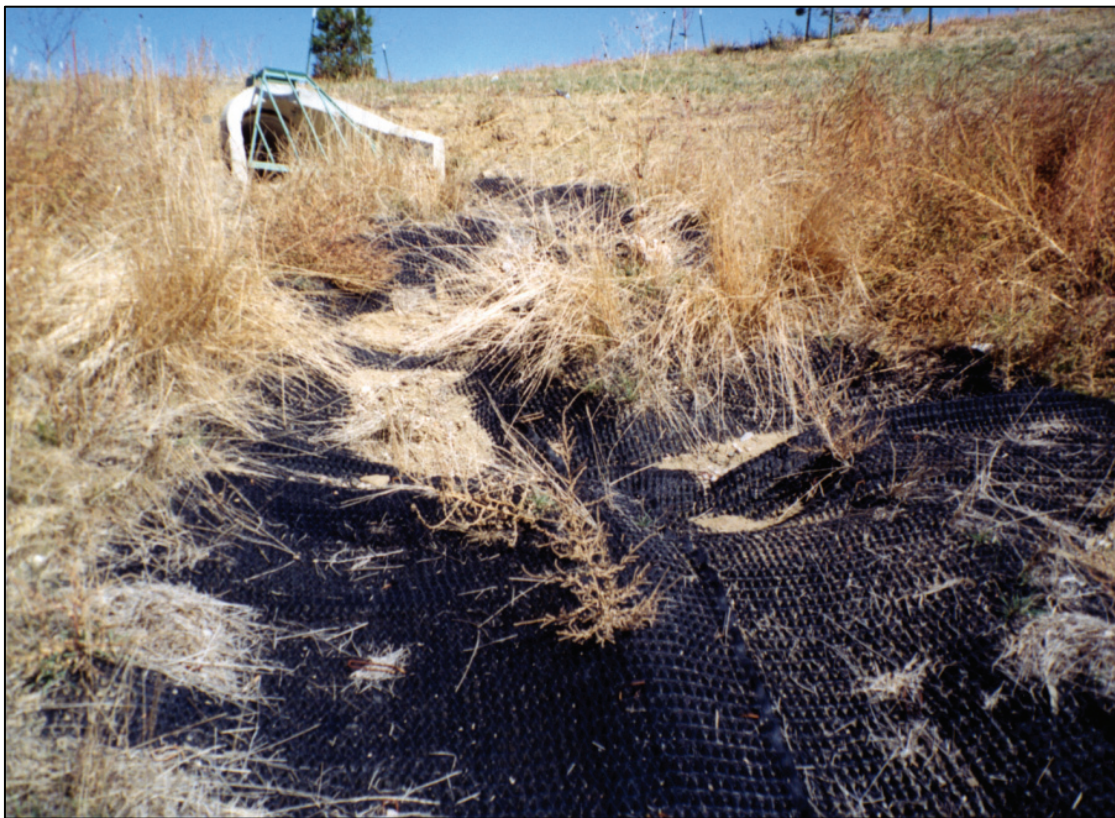
Photograph HS-15—A failed rundown that relied upon a geotextile membrane for stability.
