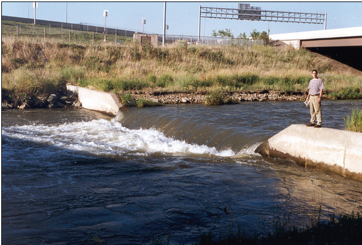
Photograph HS-2—The Clear Creek I-25 vertical concrete drop structure was a “drowning machine” until it was retrofitted by CDOT with a 10:1 downstream face. (Photograph taken before retrofit.)
