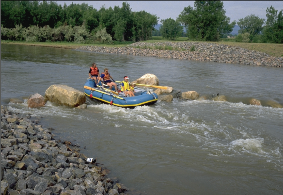
Photograph HS-16—The unsightly and hazardous 8-foot-high Brown Ditch weir was replaced with three low-head drop structures having a 10:1 downstream slope and a boat chute. The resulting improvement by the USACE has provided for safe, enjoyable recreational boating.
