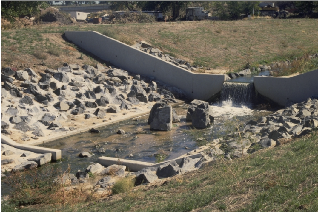
Photograph HS-8—A vertical hard basin drop structure can be an effective tool for controlling grade, but its use in urban areas is not generally recommended because of public safety concerns and aesthetics.
