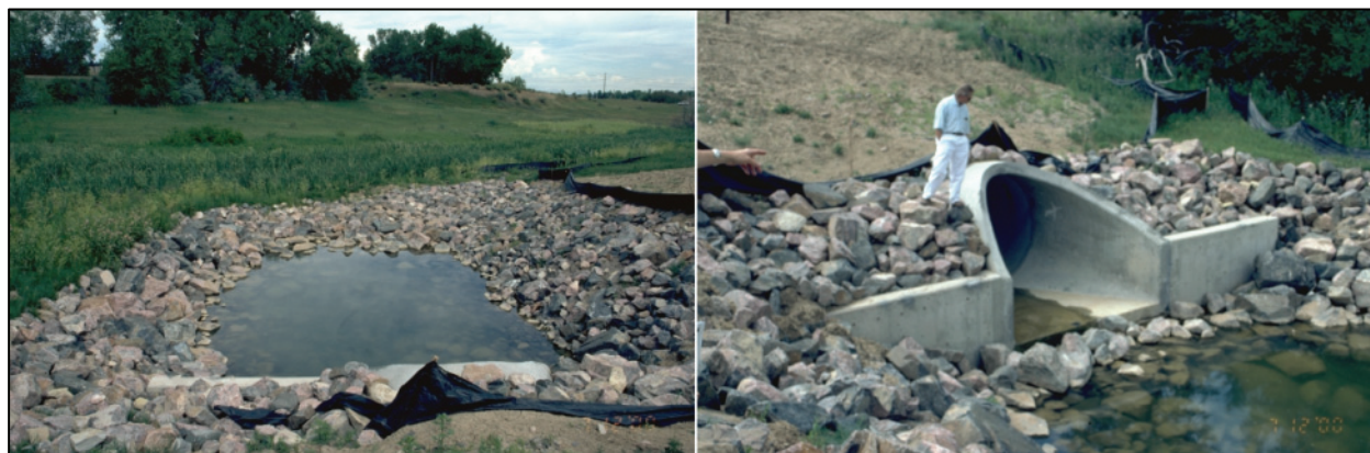
Photograph HS-12—Upstream and downstream views of a low tailwater basin in Douglas County protecting downstream wetland area. Burying and revegetation of the rock would blend the structure better with the adjacent terrain.
