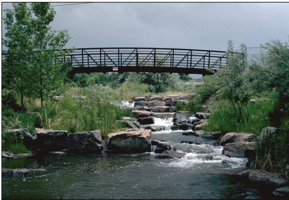
Photograph HS-7—An overall view of the drop structure from the previous page is illustrated here to emphasize the opportunities available for creating an attractive urban hydraulic setting for the riparian corridor.
