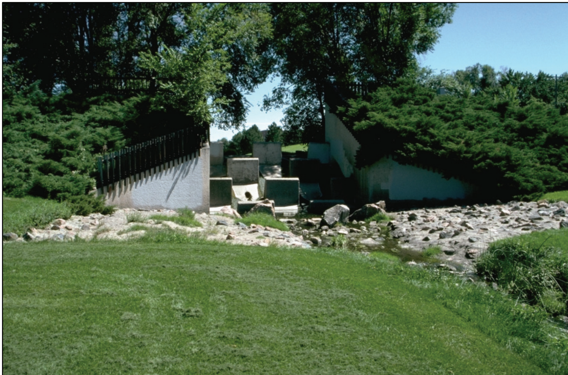
Photograph HS-1—Denver's Harvard Gulch Flood Control Project introduced the baffle chute drop structure to urban flood control in 1966. Vegetation and time have made the structure part of the city's urban poetry.
