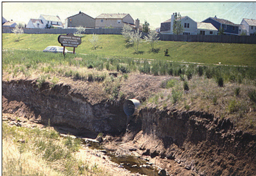
Photograph HS-11—Unprotected urban channels can experience bank erosion and degradation when established design criteria are not used. The invert of pipe used to be at invert of channel before degradation occurred.
