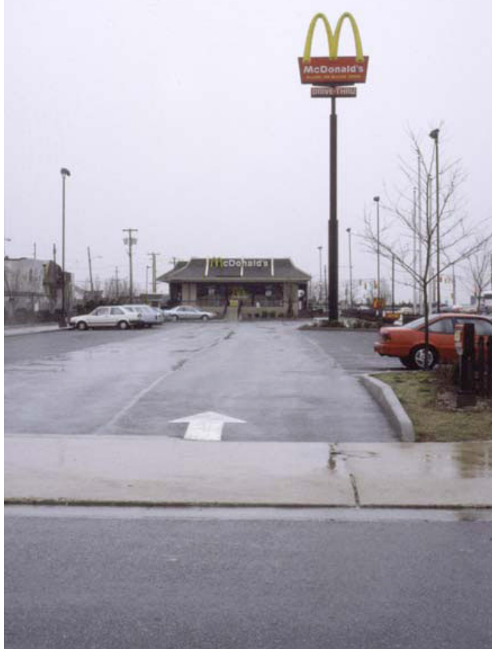
Atlantic City, New Jersey, McDonald's: pervious pavement light commercial parking lot with recharge beds.
