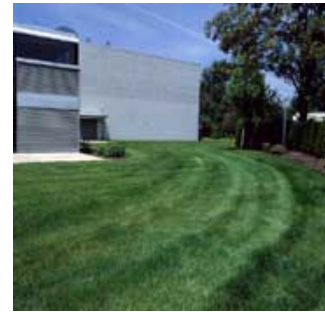
Portland Trailblazers Basketball Facility Tualatin, Oregon, Grasspave 2 Firelane
