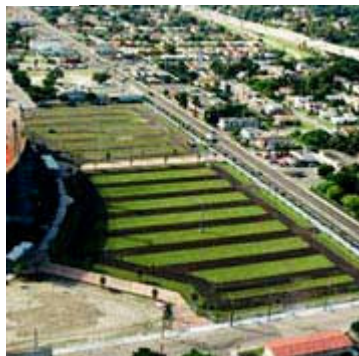
Orange Bowl Stadium Miami, Florida, Grasspave 2 Parking Lot
