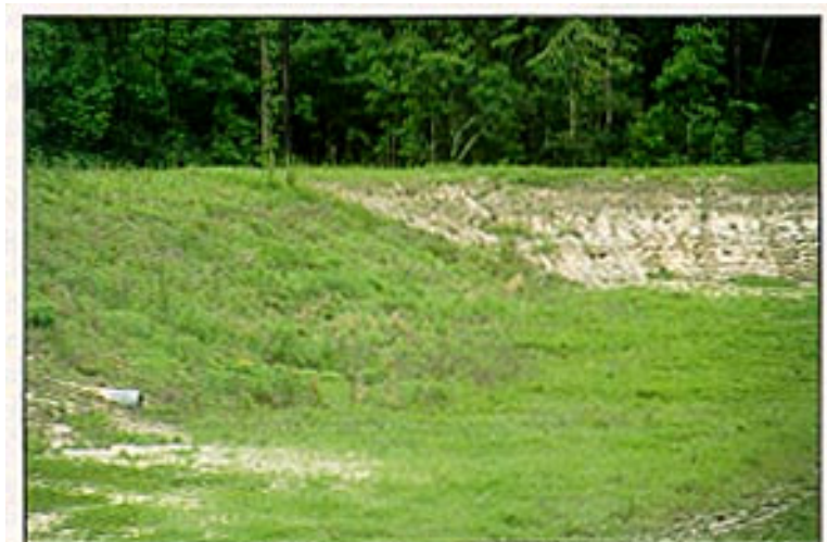
The same area on the Oaks of Terra Nova West detention basin 3 years later. Note the heavily riffled, sparsely vegetated embankment to the right of the compost area.
