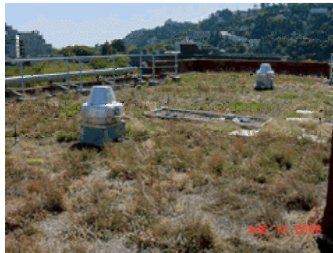
A green roof in Portland, Oregon
