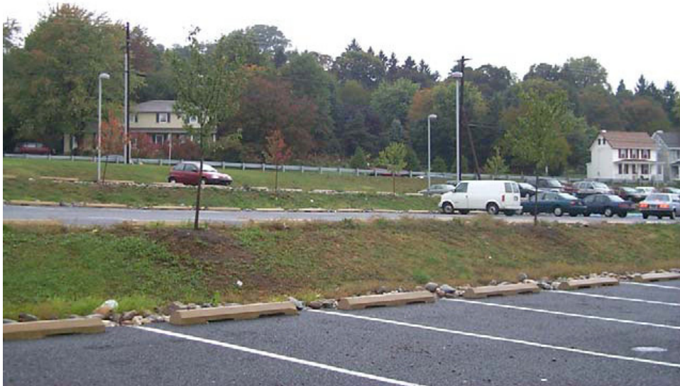
Hockessin, Delaware, City Library: pervious pavement parking lot with gravel-filled recharge beds underneath.
