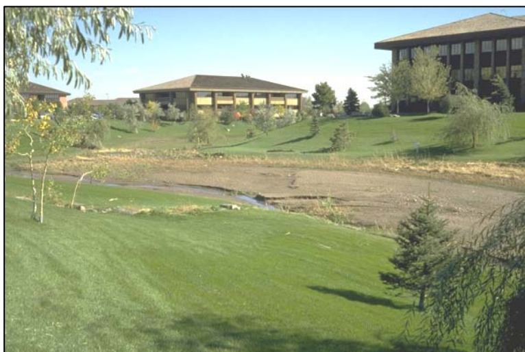
Photograph SO-8—Maintenance considerations must be carefully accounted for during design, with sediment accumulation a particular concern.
