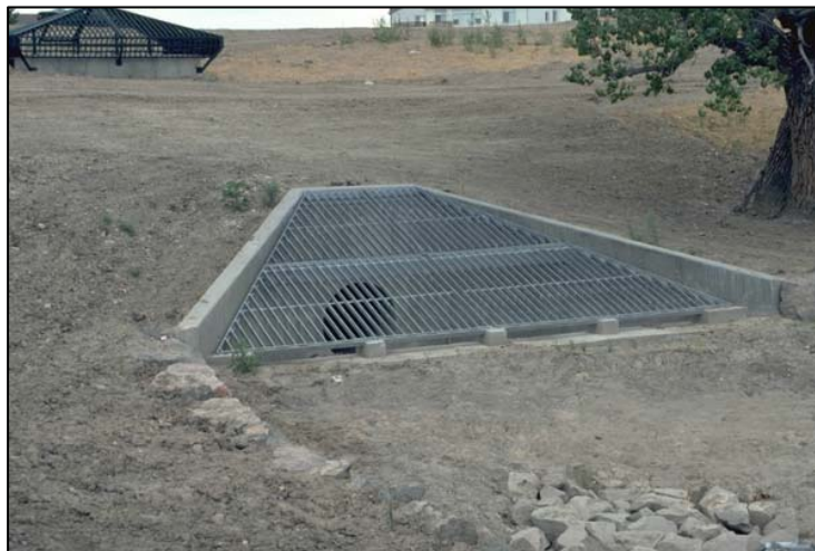
Photograph SO-6—Public safety is an important design consideration for detention facilities, including the potential need for safety/debris racks on outfall structures, as shown in this dry pond.
