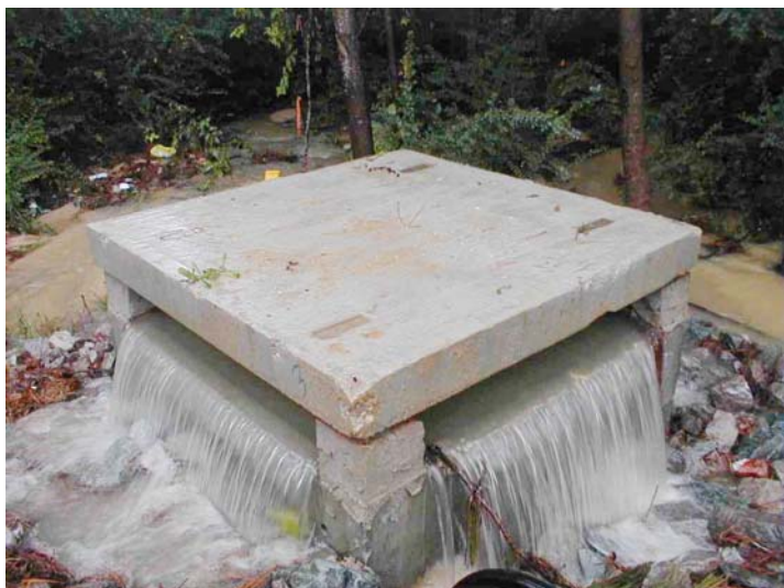
In Aberdeen, NC, a compact weir releases water on all sides, distributing stormwater to bioretention cells.
