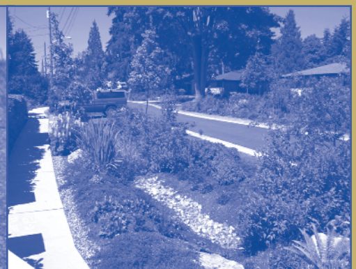
Direct runoff from pavement and buildings to vegetation-lined channels.
