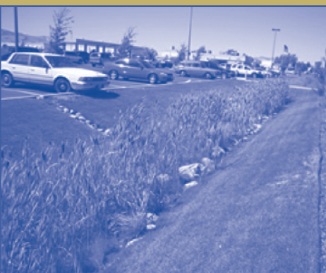
Direct runoff from pavement and buildings to vegetation-lined channels.
