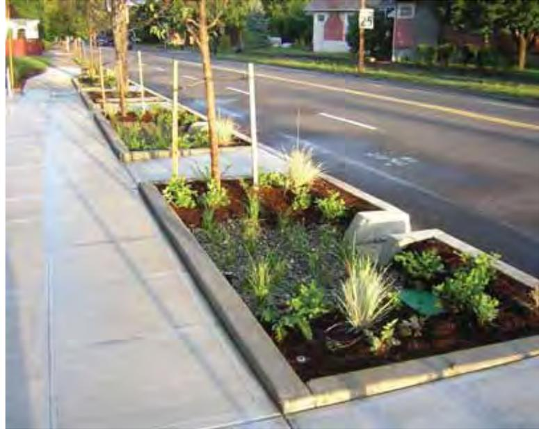
Bioswales on Portland’s Division Street infiltrate and treat stormwater runoff.
