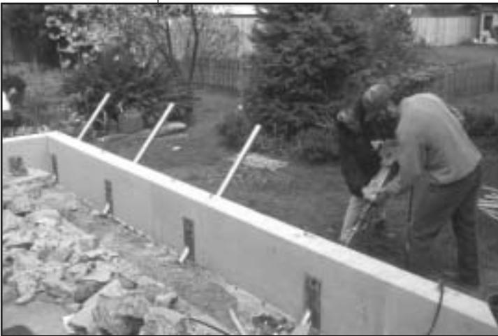
Homeowners in Olympia install a Low Impact Foundation Technology (L.I.F.T.) system as an alternative to a conventional foundation.
