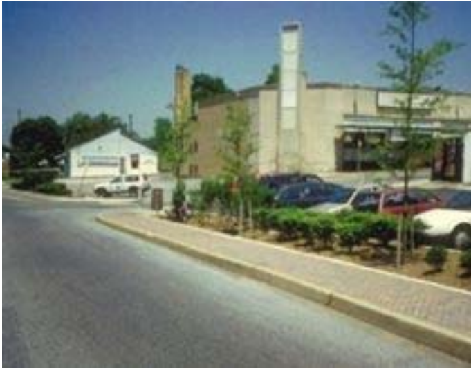
Bioretention incorporated into shopping center retrofit. Source: LID Center
