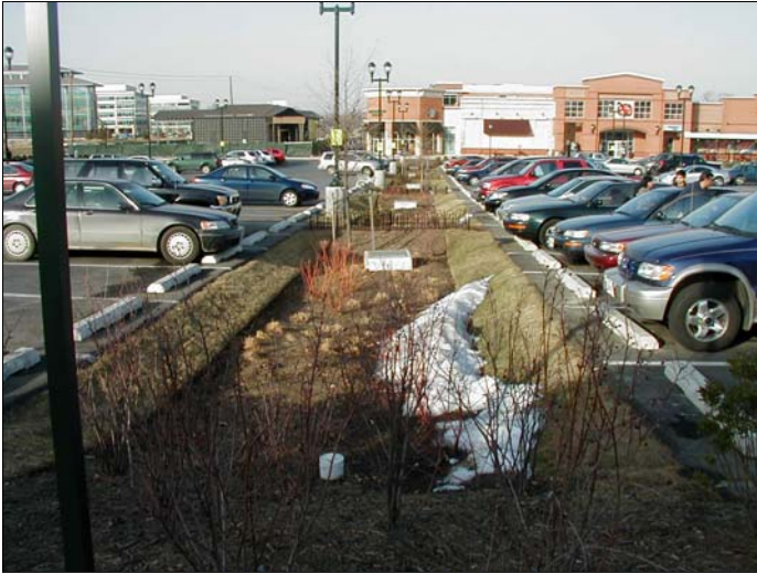
Bioretention cell in a commercial parking lot Source: LID Center, Inc
