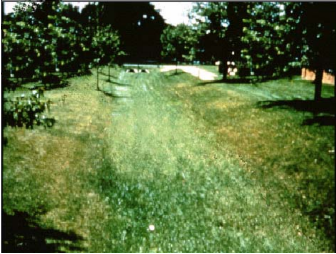
Grassed Swale Source: I ID Center
