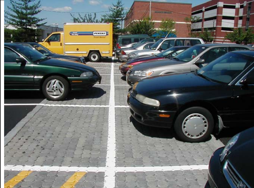
Washington Navy Yard Bldg 166 Completed ◆ Permeable Pavement
