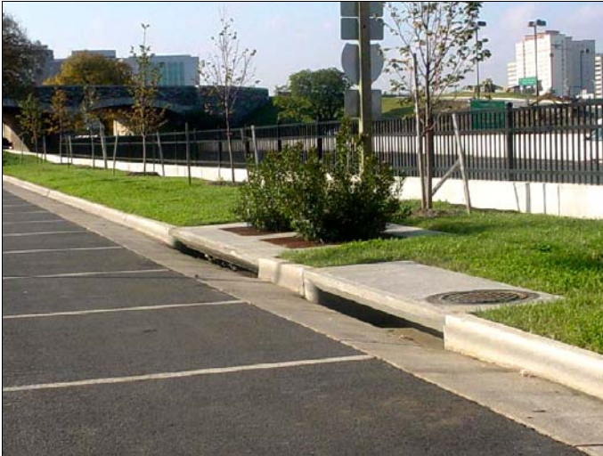
Tree box filter at the Pentagon Source: LID Center
