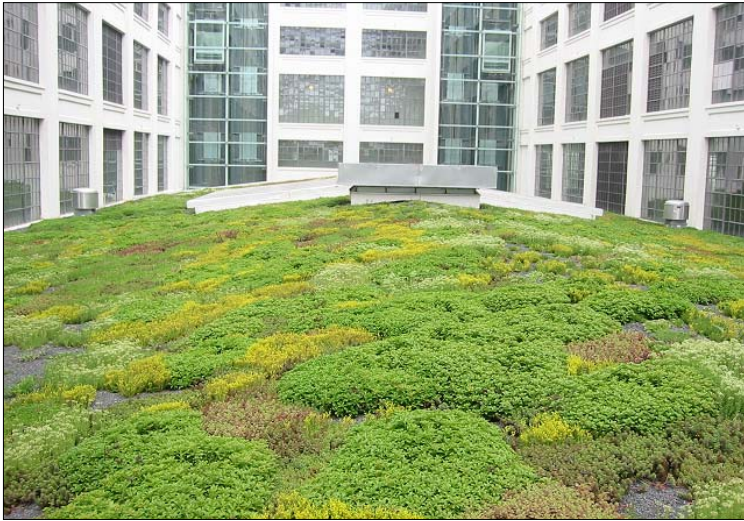
Extensive green roof in Baltimore, MD Source: Katrin Scholz-Barth Consulting.
