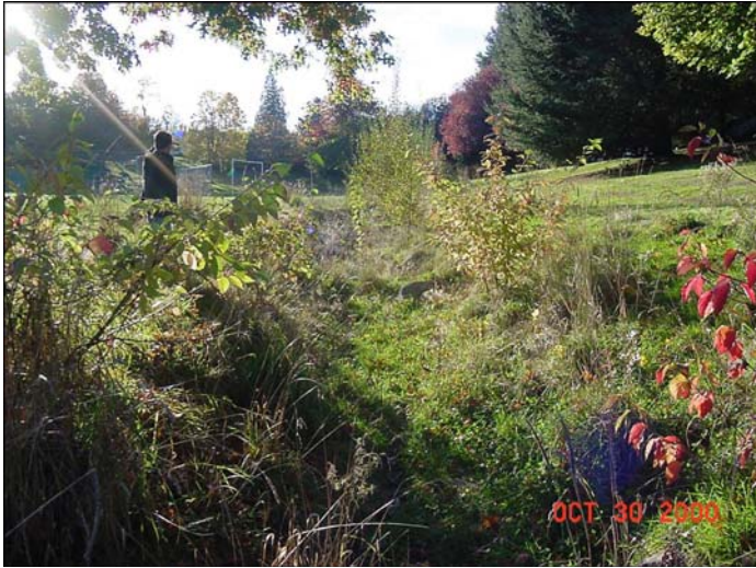
Bioretention Swale Source: Portland BES
