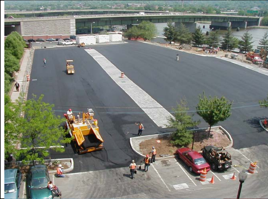
Washington Navy Yard Bldg 166 Under Construction ◆ Permeable Pavement
