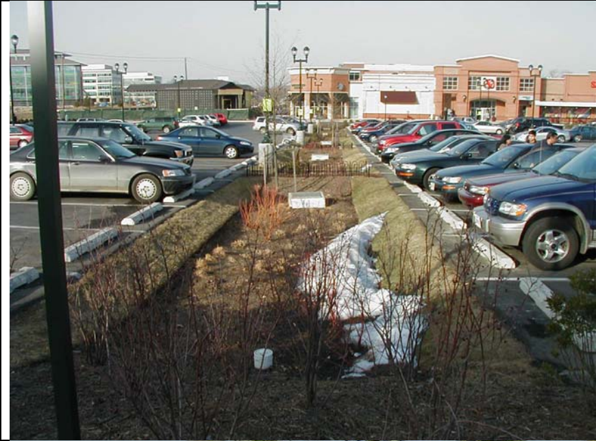
Safeway Parking Lot ◆ Bioretention
