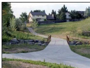
Photo 3. New Grouted Boulder Structure & Pedestrian Bridge
