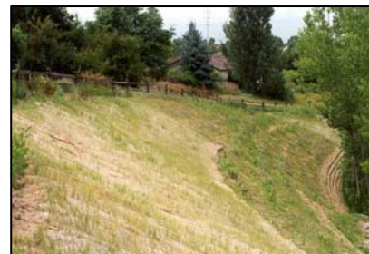
Photo 7. Completed Slope with Brush Layering, Erosion Mat, and Wrapped Soil Lifts
