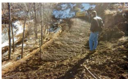
Photo 6. Construction of Brush Layering
