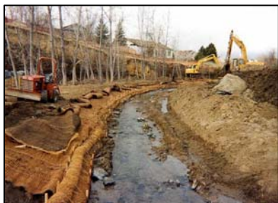
Photo 4. Biolog & Erosion Mat Installation
