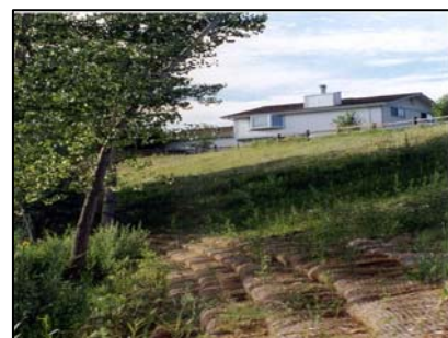
Photo 5. Reconstructed Slope with Wrapped Soil Lifts at Toe
