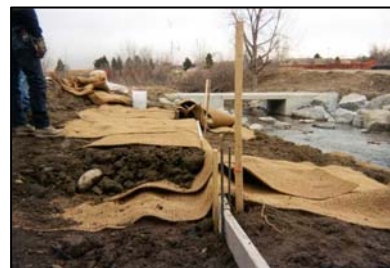
Photo 9. Construction of Wrapped Soil Lifts
