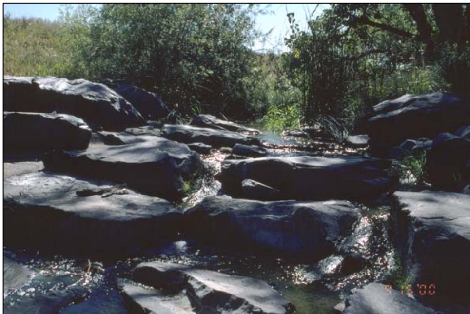
Stream Bank Stabilization Including Grouted Boulder Check Structure With Low-Water Crossing, Slope Flattening, And Revegetation
