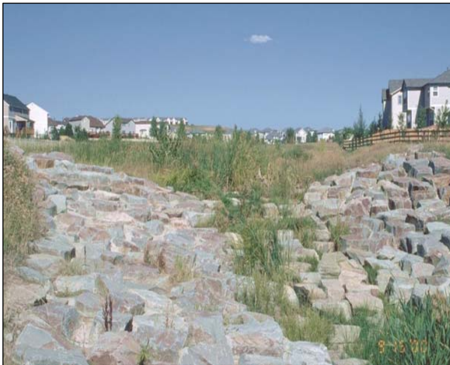
Grouted Boulder Drop Structures on Tributary LB-3 Channel
