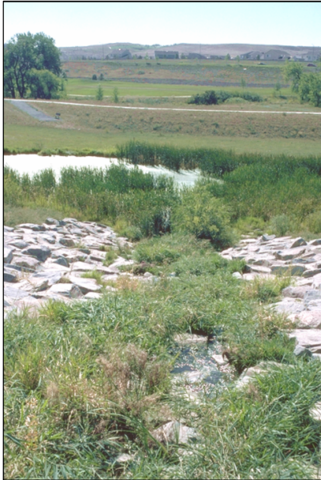
Grouted Boulder Drop Structures on Tributary LB-3 Channel
