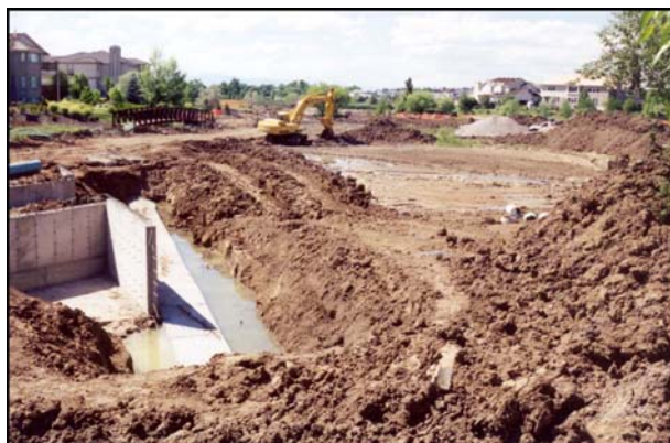
Photo 6 Excavation of Accumulated Sediment
