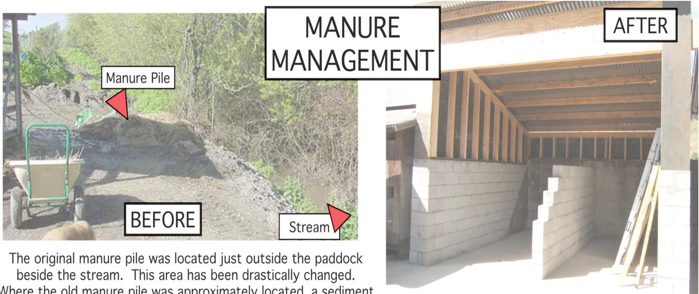
The original manure pile was located just outside the paddock beside the stream. This area has been drastically changed. Where the old manure pile was approximately located, a sediment basin has been constructed. This area is a small depression that detains the outlet from the drains and allows the sediments to filter out before the clean water is released near the stream.
