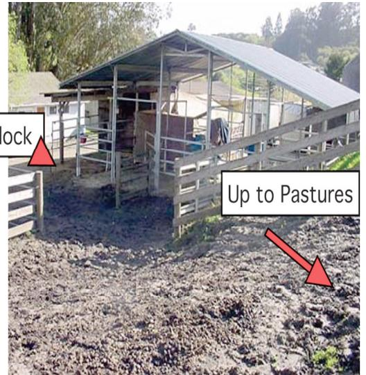
Because the barn and paddock were located at the base of the hill, all of the water that fell on the slope would flow down and collect there. This meant that as you got closer to the barn the muddier it became.
