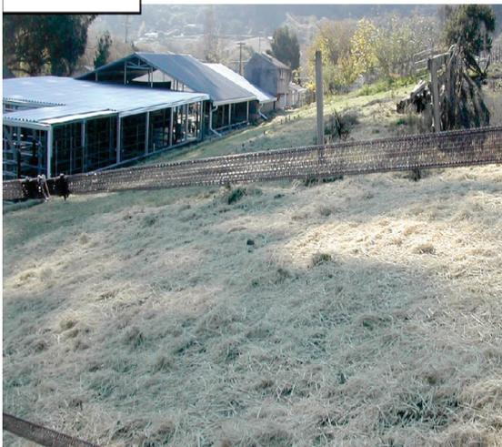
Once the wall was built and the drains were installed the paddock was ready to be regraded and resurfaced. The wall, drains and vegetation will manage the runoff so that the paddocks will stay dry. To add one more layer of protection, the owners erected a roof over their paddock and installed gutters which empty into the French Drain.
