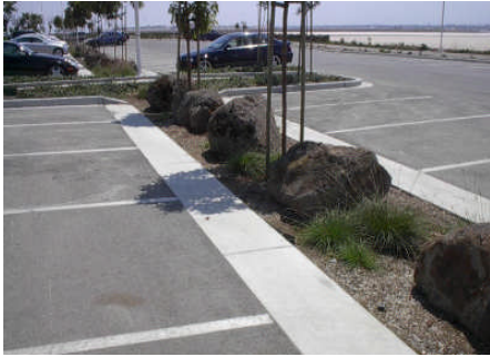
Figure 2. A parking lot island that allows for storm water infiltration is an example of a LIP BMP.
