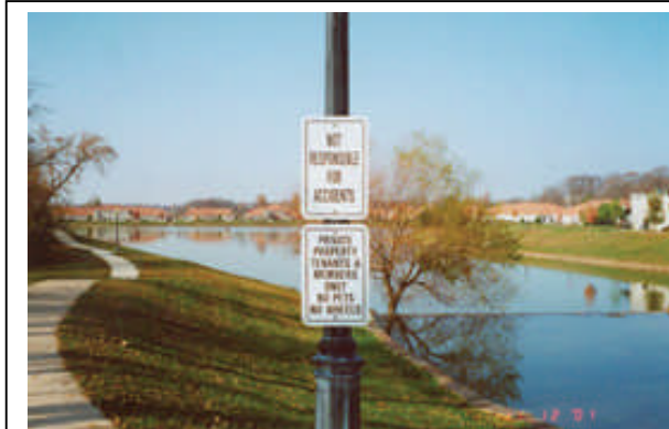
Figure 7. Signs posted around wet ponds warn the public about the nearby danger of open water.
