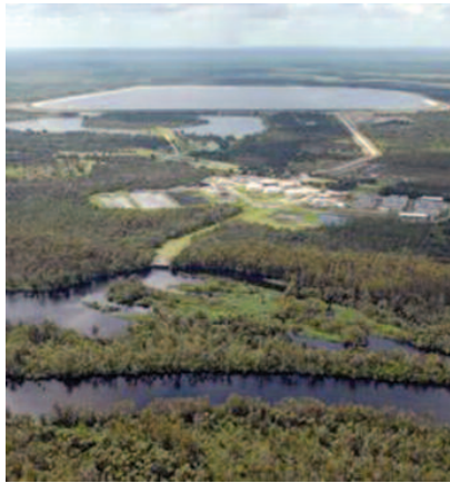
Photo courtesy of Peace River Manasota Regional Water Supply Authority.
