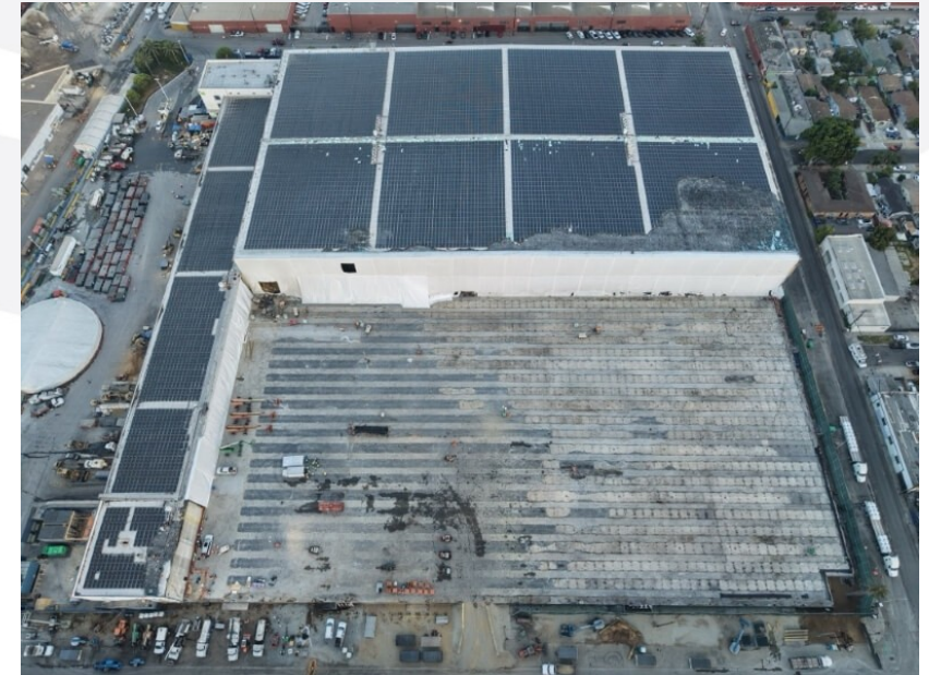
Lineage's Los Palos Street facility as of August 10 th . Photo retrieved on September 17, 2026 from Lineage's website at https://www.onlineage.com/boyle-heights-fire-response
